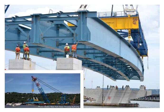
**THE FIRST MASSIVE SECTION OF** structural steel for the approach span of New York's new Tappan Zee Bridge was successfully installed recently using the "I Lift NY" super crane.
