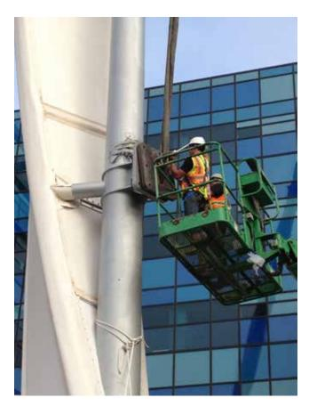
Workers prepare spire connections and templates to be attached to the building support beams.
