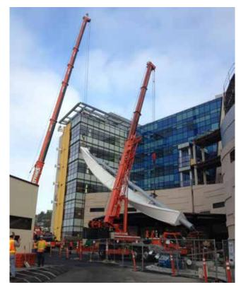
Interface between the spire and the main building came in the form of double-end plate-type connections with 2½-in. end plates and high-strength bolts.
