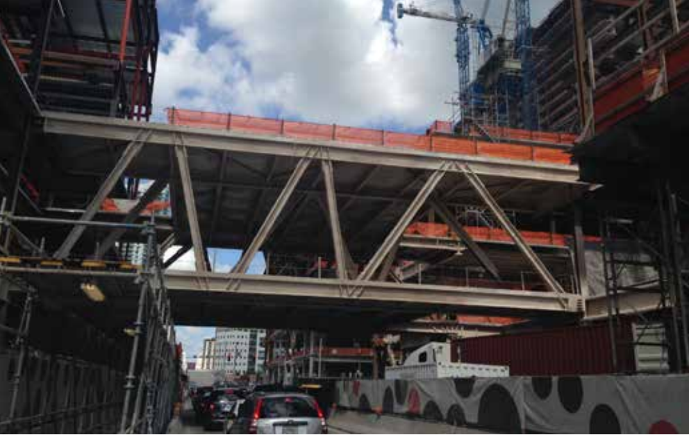
◀ The east-to-north pedestrian bridge over the roadway through the complex.
