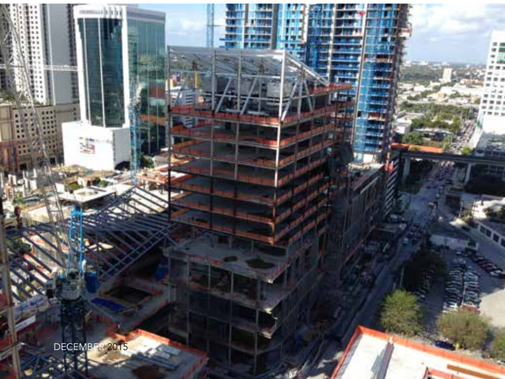
▲ Laydown area was at a premium and required load-listing the delivery trucks for steel to be used that day only.
