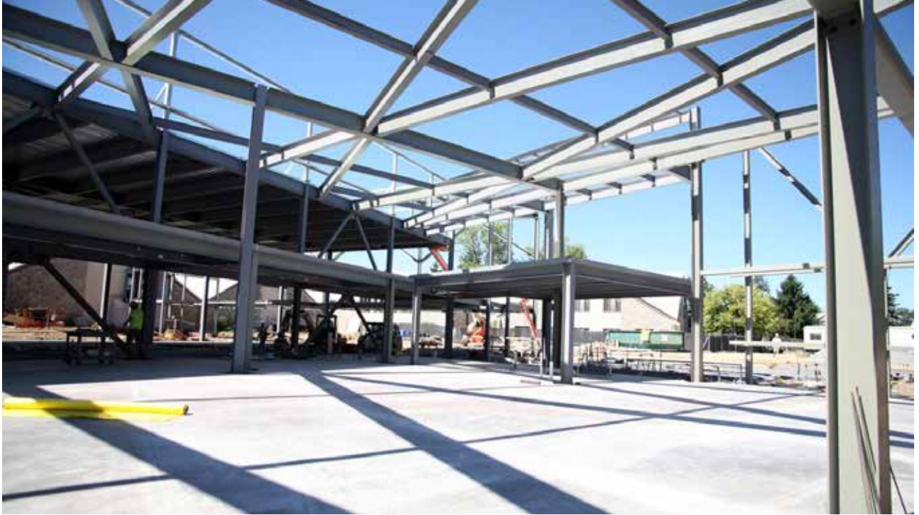
▲ Framing for the roof.
