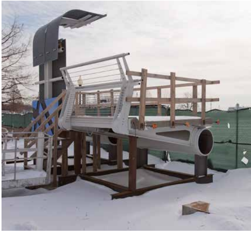
▲ A full-scale mockup of the spine, deck and railings was constructed on-site to refine the details.
