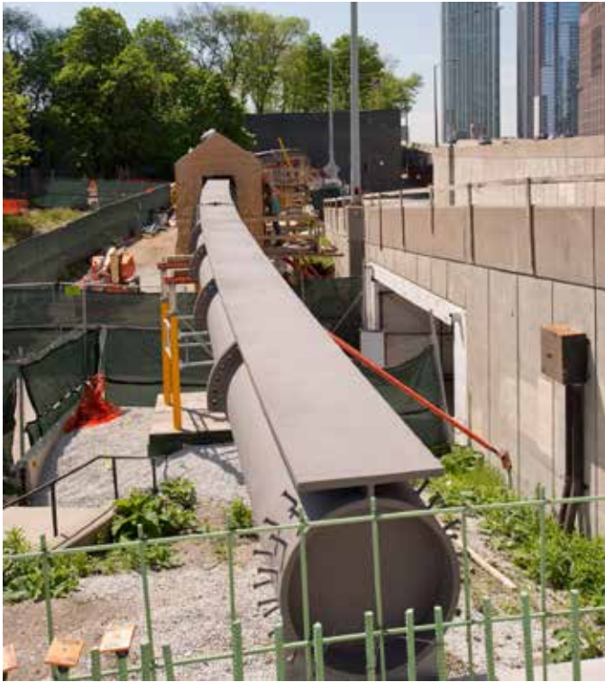
▲ ▼ The bridge's central spine is fabricated from 30-in.-diameter steel pipe, either 1¼ in. or 1¾ in. thick depending upon span and strength requirements.
