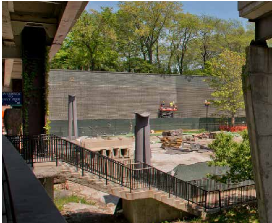
▲ ▼ The flyover spine is supported by steel columns created from 1¼-in. steel plate bent into a 30-in. by 22-in. elliptical shape along the main alignment and by cantilevered concrete abutments at its ends. At three locations, the path is supported directly from the existing bents of Lake Shore Drive.
