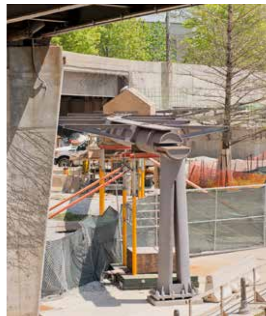
▼ The paint system is not the typical zinc/epoxy/urethane system used on highway bridges, but rather a three-coat system comprised of a primer, an intermediate coat and a fluoropolymer finish coat. Typically used on building applications, this system is highly durable and provides enhanced color and finish retention.
