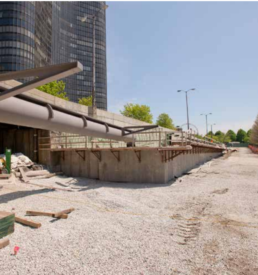
▲ ▼ The bridge's central spine is fabricated from 30-in.-diameter steel pipe, either 1¼ in. or 1¾ in. thick depending upon span and strength requirements.
