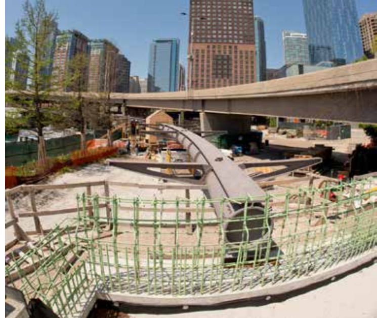
▲ The design uses the frame action created by the spine-column rigid connection. This not only controls in-plane bending, but also resists out of plan bending and torsion in the spine.
