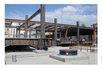
↑ The superstructure frame is supported on an energydissipating seismic isolation system above the lowest mat foundation level. This system in made up of 69 triple concave-friction pendulum (TC-FP) bearings.
