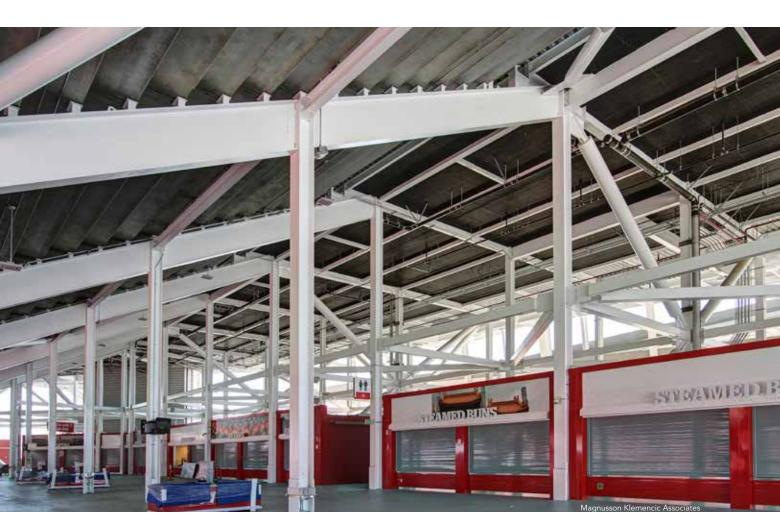
▲ The BRBs range in capacity from 100 kips to 1,800 kips and are arranged in U-shaped "brace cores" around concessions and other areas.
