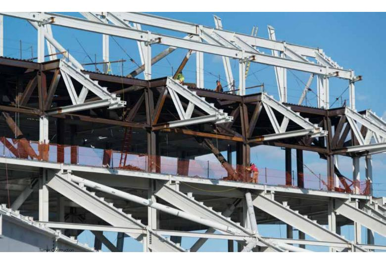
were in review, saving more than two months in terms of project delivery. In addition, the stadium was designed as four separate structures to facilitate simultaneous four-quadrant construction versus more traditional (and lengthier) "racetrack" sequencing. Ultimately, construction of the stadium took just 28 months, starting in April 2012 and finishing in early August 2014, in time for the kickoff of the NFL season.
