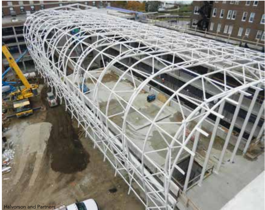
▲ ▼ Bender-Roller Chicago Metal Rolled Products used a three-roll, pyramid bending process to curve the 36 tons of HSS to various radiuses from 250 ft to 12 ft.
