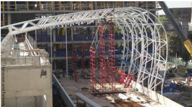
▼ Erecting the HSS framing for the Winter Garden.
