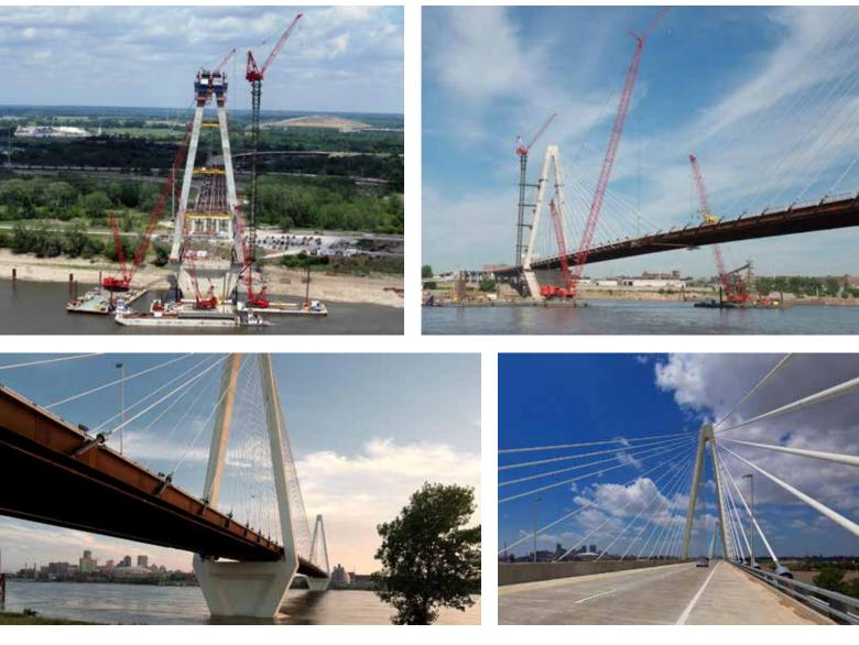
The superstructure was designed to be redundant and able to withstand the loss of any cable without significant damage to the bridge. The cable spacing was optimized to assist with the load transfer in the superstructure under the cable-loss scenario. Various details were incorporated into the design of the bridge to address security measures important in today's world.
