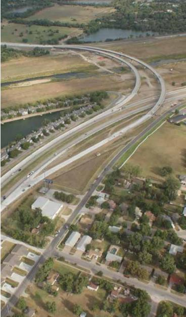
bridges' horizontal curvature and span lengths up to 225 ft, and weathering steel was selected to minimize future maintenance requirements. In all, the bridges use 2,875 tons of structural steel.
