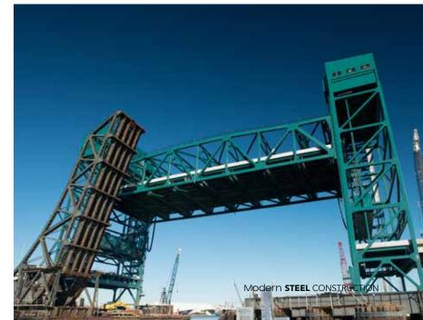
Because rock was too deep to rest the drilled shaft foundations on, the foundations were predicted to experience some settlement with time. Settlement can be an issue for any bridge, but is of particular concern for movable bridges because of the precise tolerances required to ensure operation without binding. Jacking brackets were designed into the towers to allow them to be jacked under full, dead load to compensate for the settlement.
