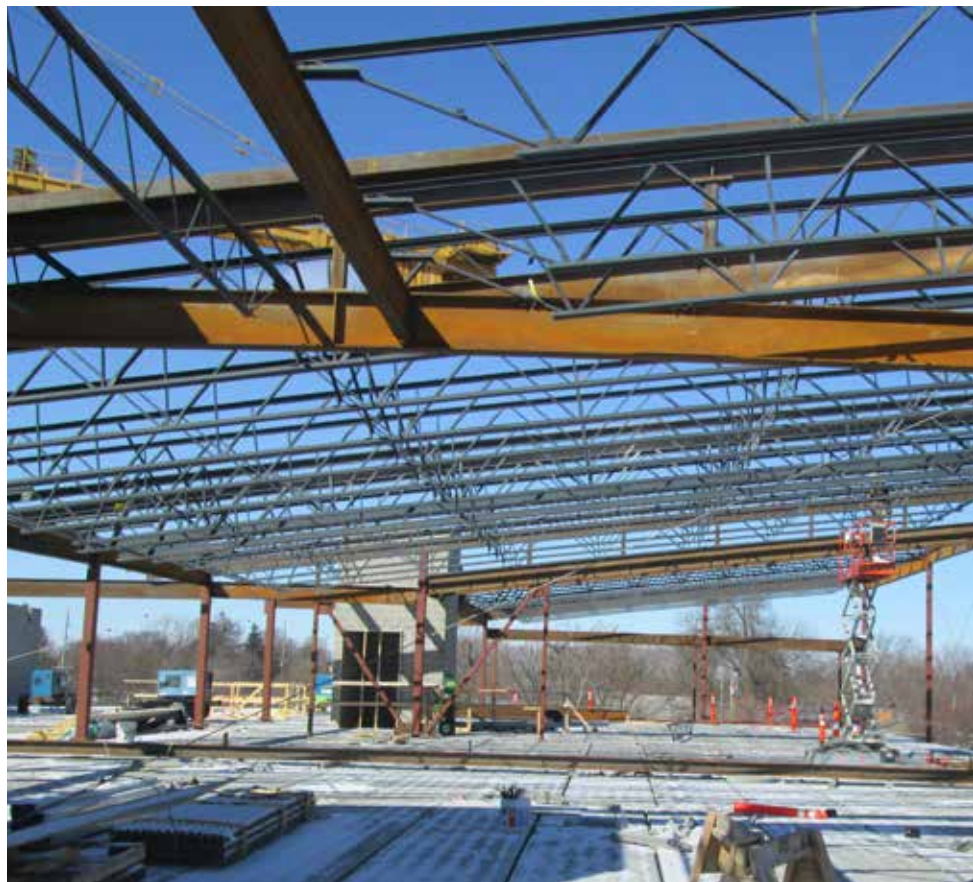
▲ The steel framing for the 112-ft-long skywalk facilitated a 7-ft horizontal bend and a 2-ft elevation change between the existing facility and the new addition.
