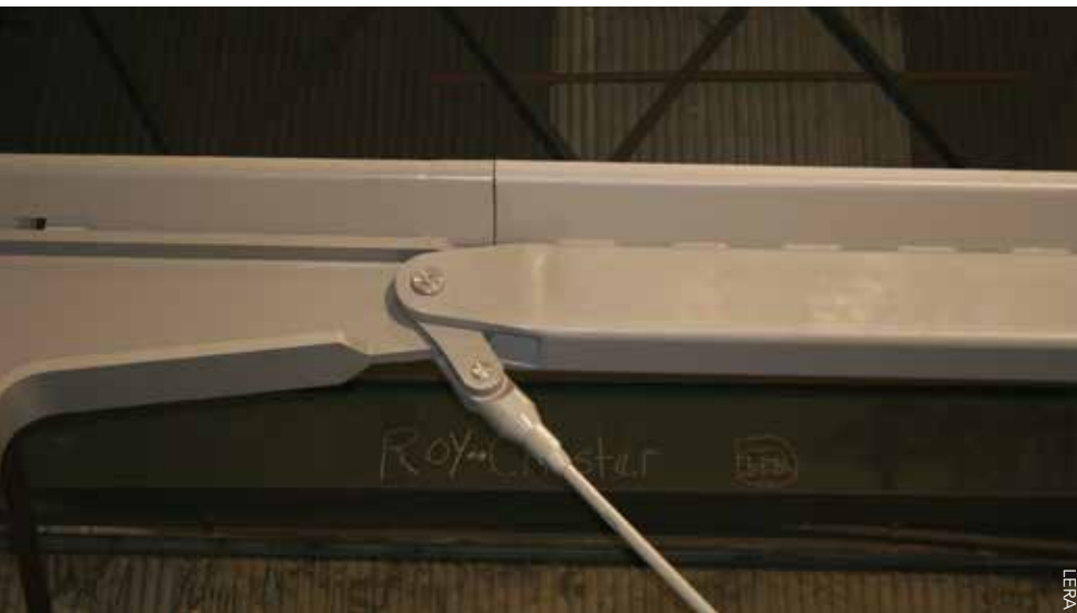
▲ Close-up of an AESS pin.
