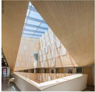
Two existing open bays at the center of the original penthouse floor/low roof form the basis for the light well, which extends up through the new fourth floor and roof.
