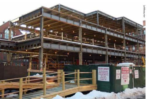
▲ To stiffen the building against wind loads in both directions, the team developed two special bracing systems that responded to both the new architecture and the existing framing.
