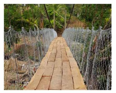
▲ ▼ The bridge was made of local materials consisting of custom bent rebar suspenders with steel cross-beams, timber decking and safety fencing.
