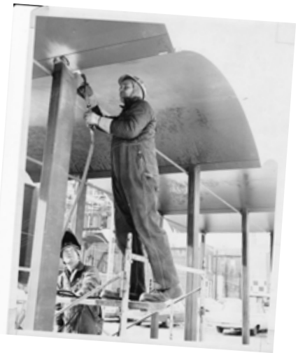
▲ Michelmann ironworkers on the job.
