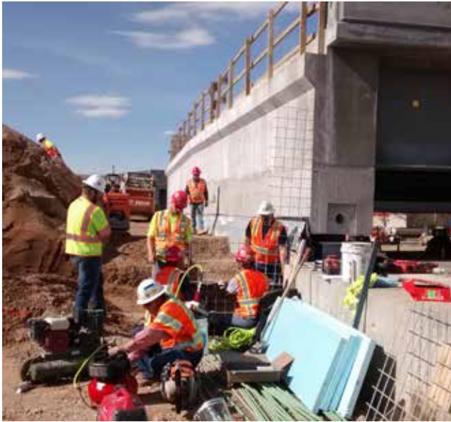
▲ Wing wall construction, following the slide.
