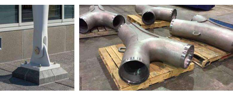
A universal pin connector with an architectural taper.
