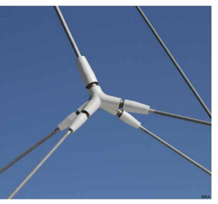
A closeup of a single turnbuckle casting on the San Ysidro Land Port of Entry project. effective solution. Experienced casting suppliers can offer insight on how the freedom of geometry offered by castings can best be leveraged to address design or constructability challenges and assist the design team in understanding the value and economy—as well as attractiveness—that castings can offer to the project as a whole.
