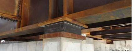
▲ Steel-reinforced bearings for acoustic and structural isolation.
