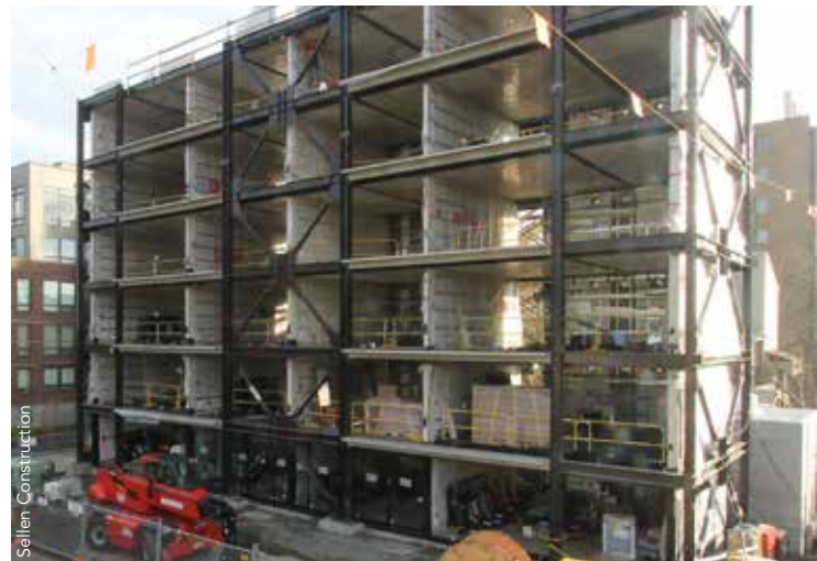
▲ ▲ ▼ The external steel gravity and lateral system allowed for an efficient design that was very quick to erect. Bolted connections were used exclusively.
