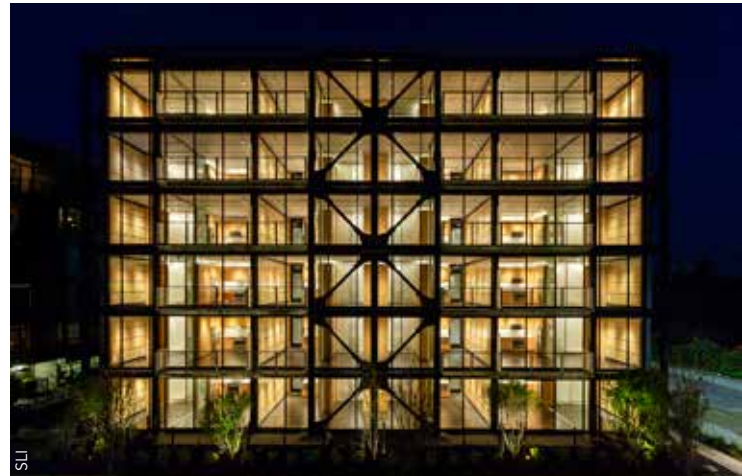
▲ ▲ ▼ The external steel gravity and lateral system allowed for an efficient design that was very quick to erect. Bolted connections were used exclusively.
