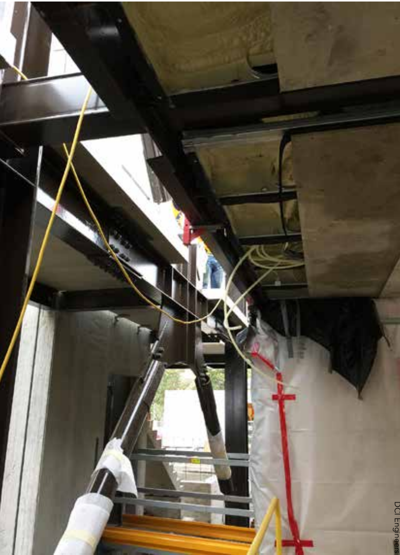
▲ ▲ ▼ The external steel gravity and lateral system allowed for an efficient design that was very quick to erect. Bolted connections were used exclusively.
