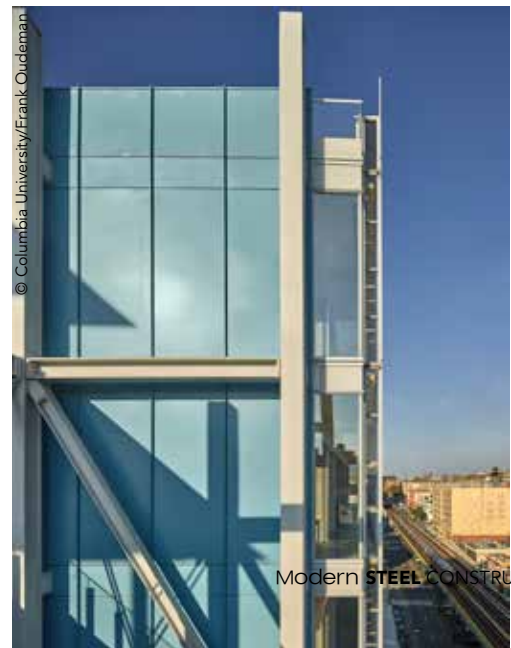
▼ Exposed exterior steel of the science center.
