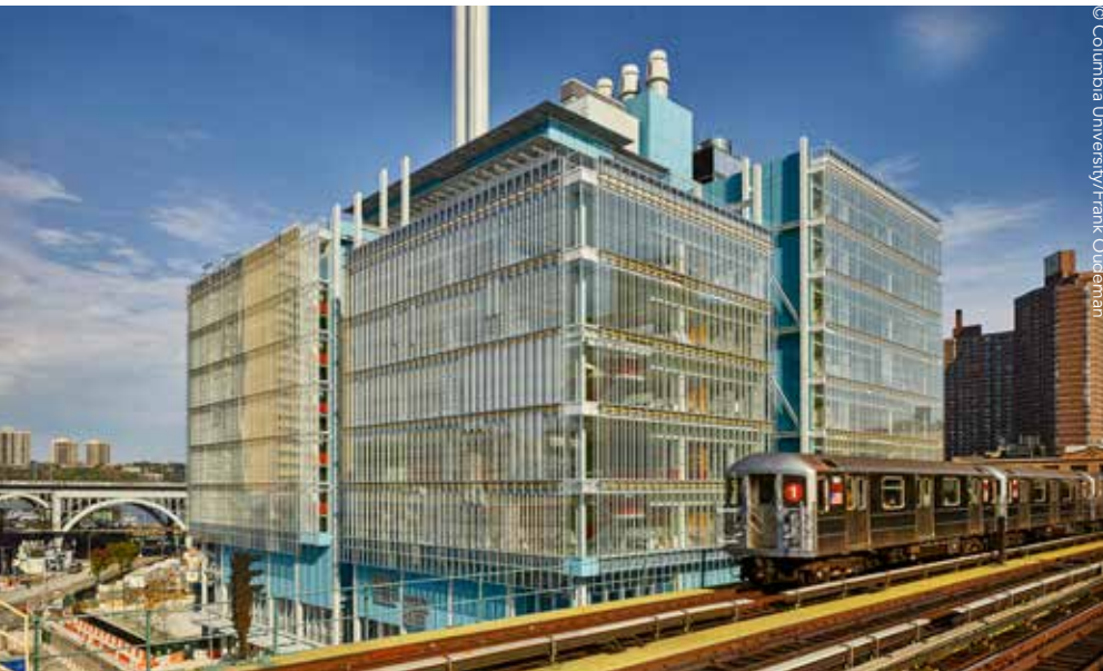
▲ Proximity to the elevated subway line required enhanced sound and vibration mitigation.
