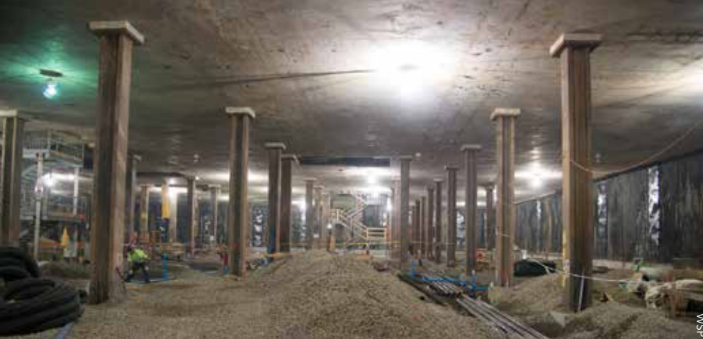
◀ Excavation during the top-down construction process.
