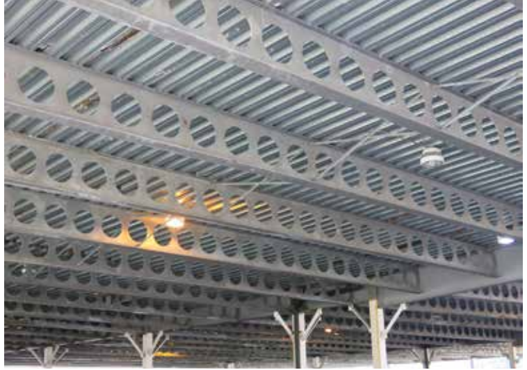
▲ Exposed beams in a parking garage project.
