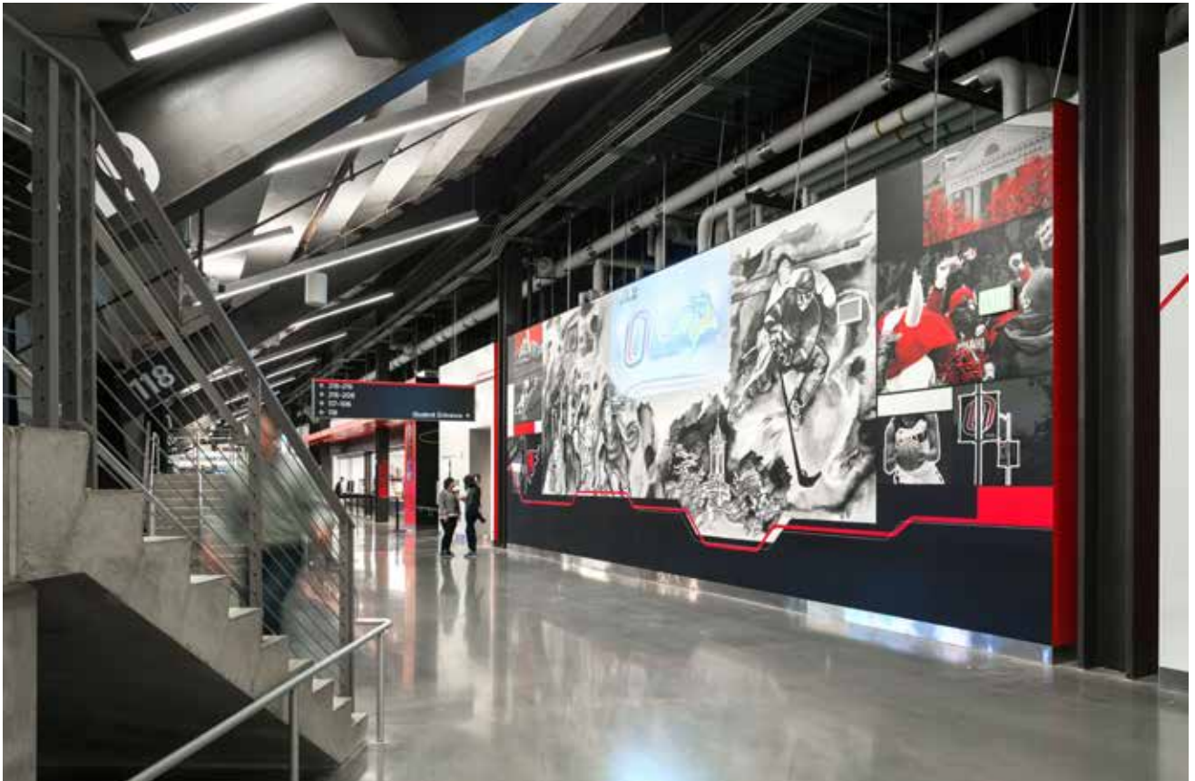
▲ One of the concourses, featuring exposed steel framing for the seating.
