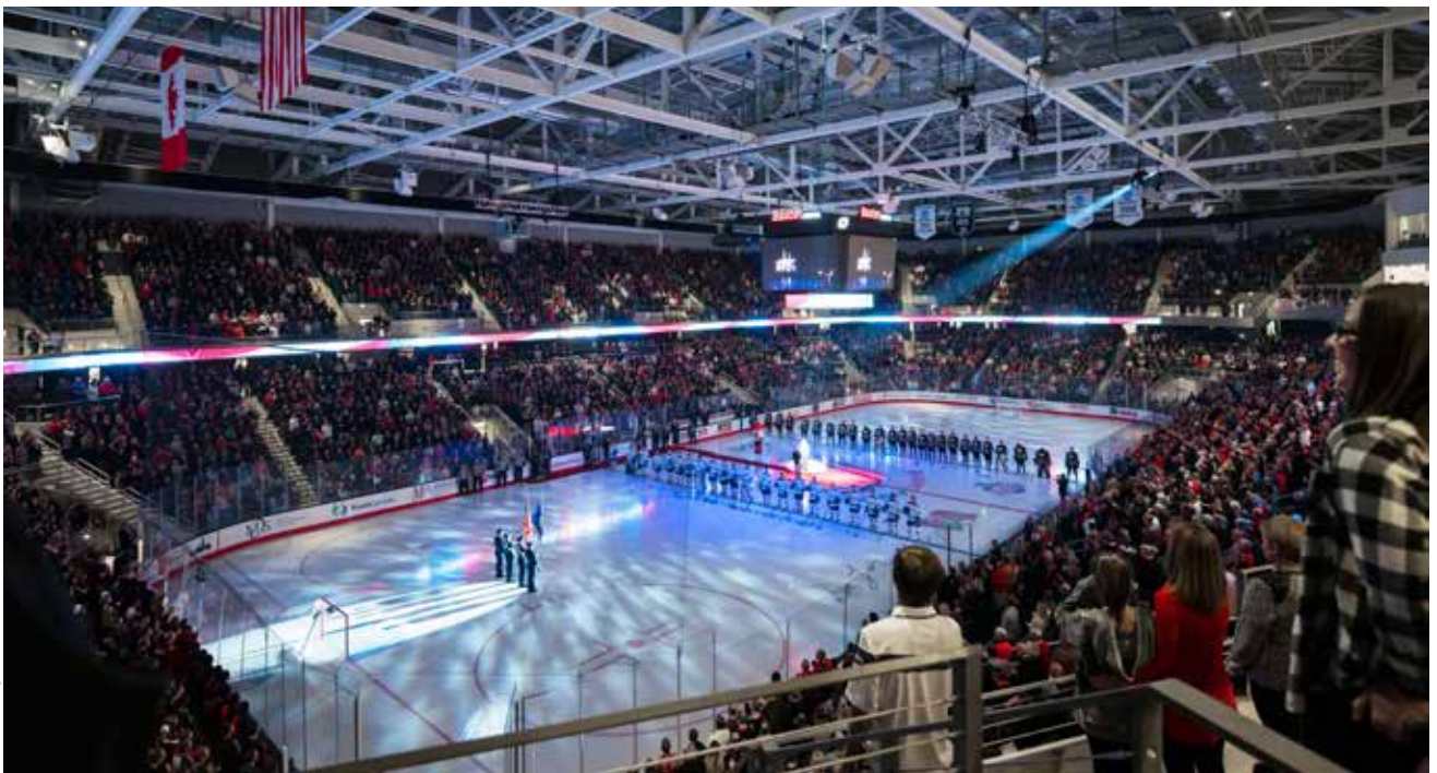
▼ The roof structure was painted white and the roof deck was left galvanized to serve as design elements.
