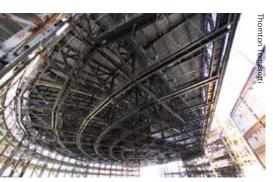
Tomasetti proposed an innovative approach that integrated temporary works to erect the 4,200-ton roof.
