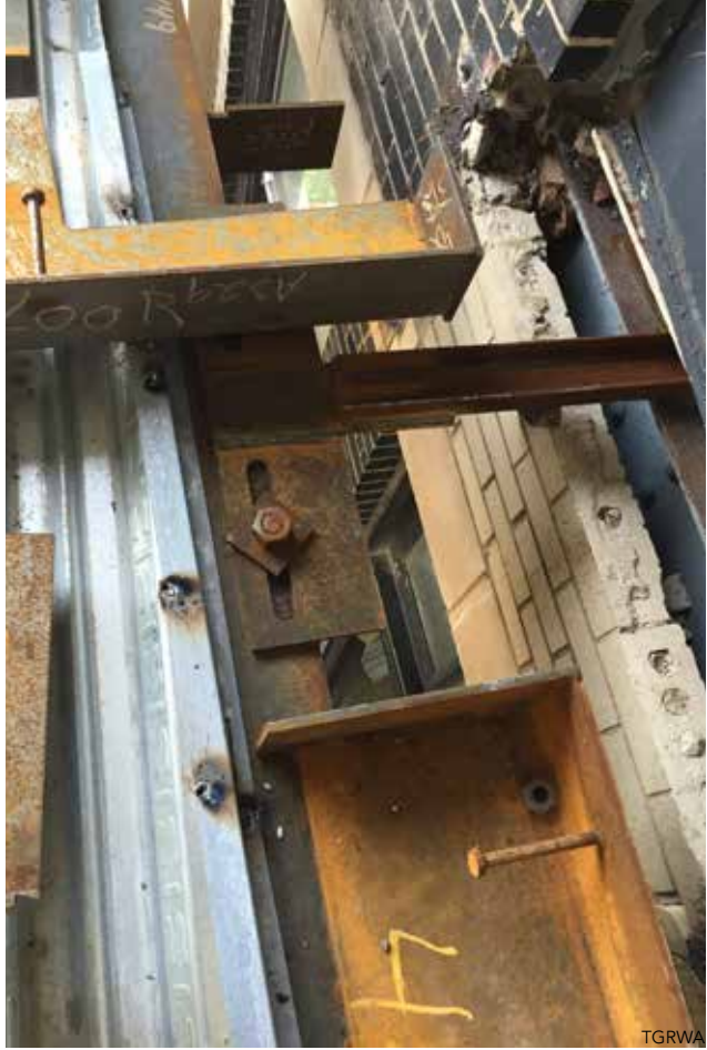
▲ Slab edge framing and attachment to the adjacent building.
