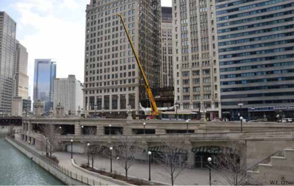
◀ Various views of the double-web plate girder erection. There are four of these girders in all, each framing to a single wide-flange column and transferring the load of the 18 floors above the ballroom level.
