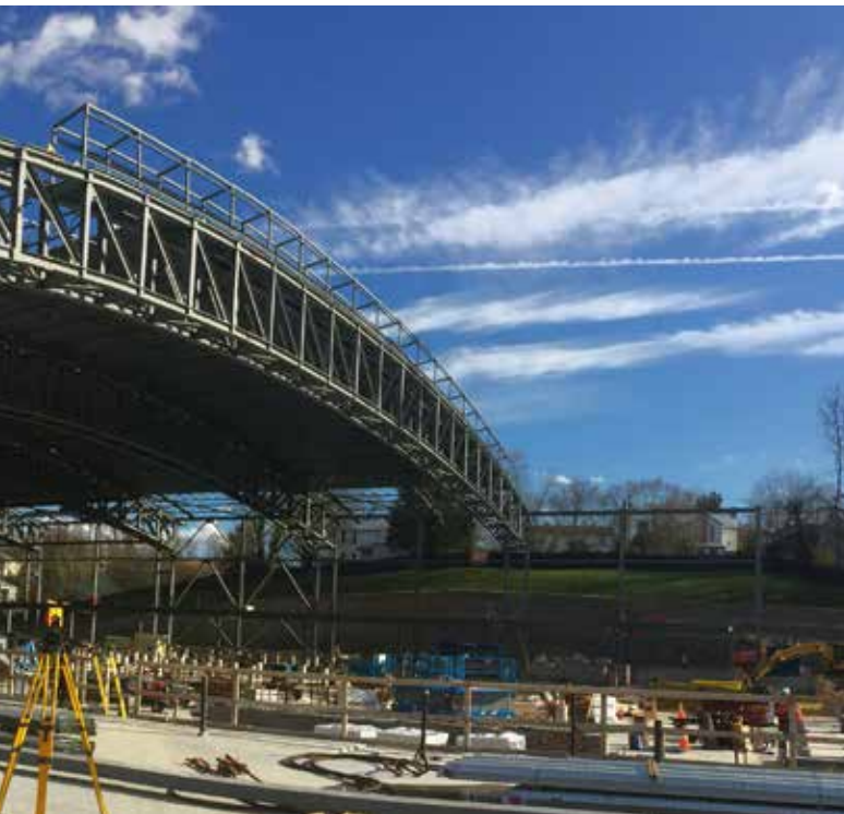
▼ A roof truss, prior to erection.
