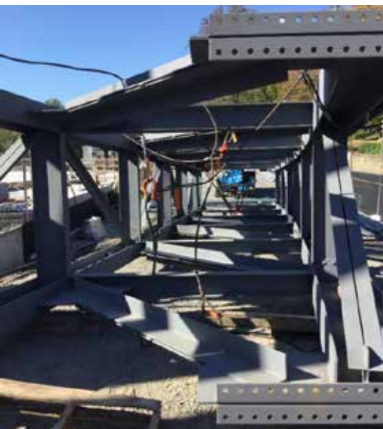
▼ A roof truss, prior to erection.
