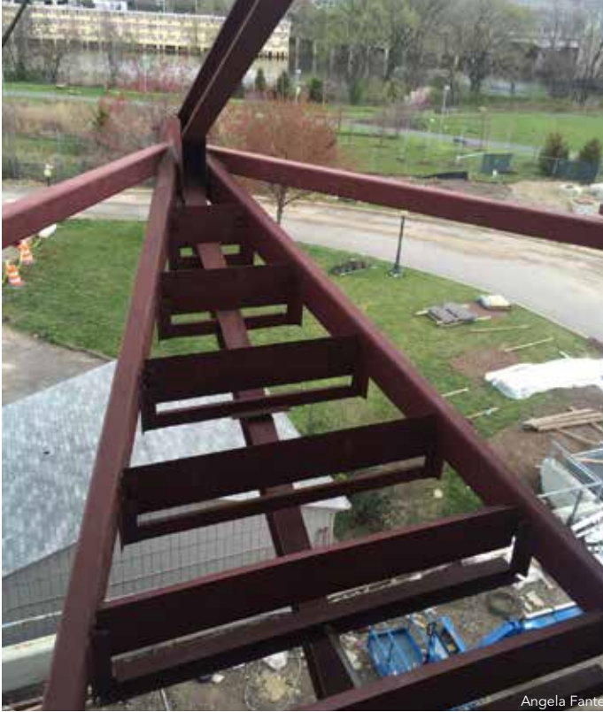
◀ ▲ Structural engineer Ballinger developed a framing concept comprised of a series of diagonal compression props/columns with corresponding tension ties at the floor levels (or vice versa) in order to minimize the new structure's weight and depth.
