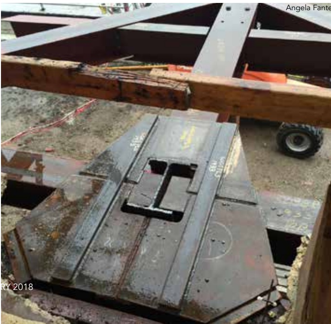
▲ The angular nature of the addition created unique interior spaces. ▼ Custom gusset plate connection plan details and sections were provided at each of the 28 distinct connection points.
