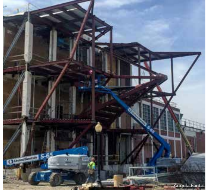
◀ ▲ Structural engineer Ballinger developed a framing concept comprised of a series of diagonal compression props/columns with corresponding tension ties at the floor levels (or vice versa) in order to minimize the new structure's weight and depth.
