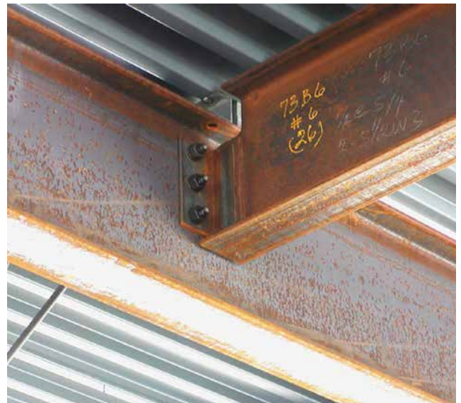
▲ Figure 1. Beam coped at the top flange.
