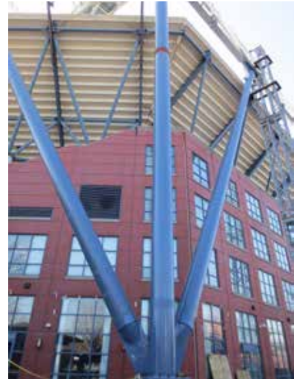
▲ Arthur Ashe Stadium in New York uses large cast connections to create a uniform look at the eight transfers.
