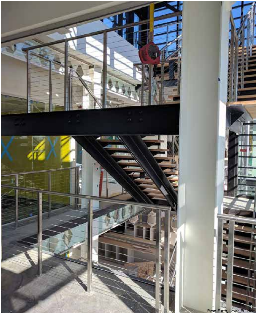
Ryan Furth, Lewis Builders
