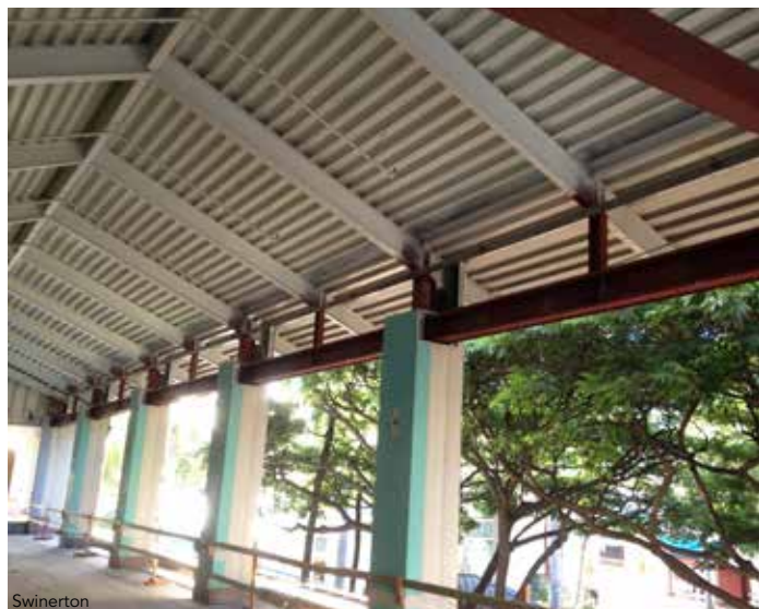
New steel-supported roof.
