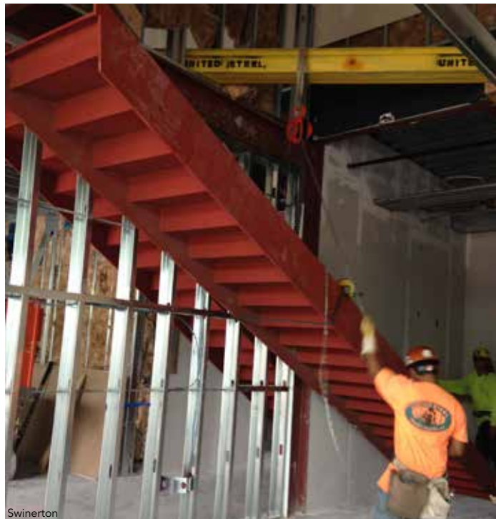
above: Steel student apartment stairs being installed... below: ...and in place following project completion.
