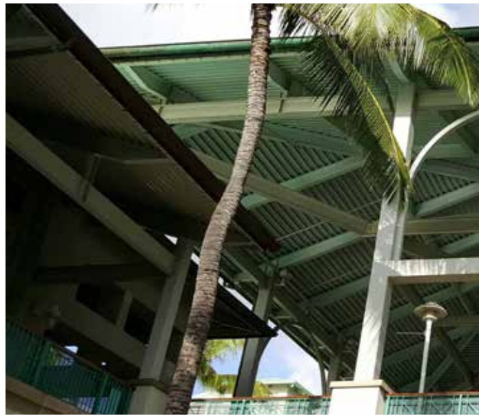
Steel roof framing and supports.
