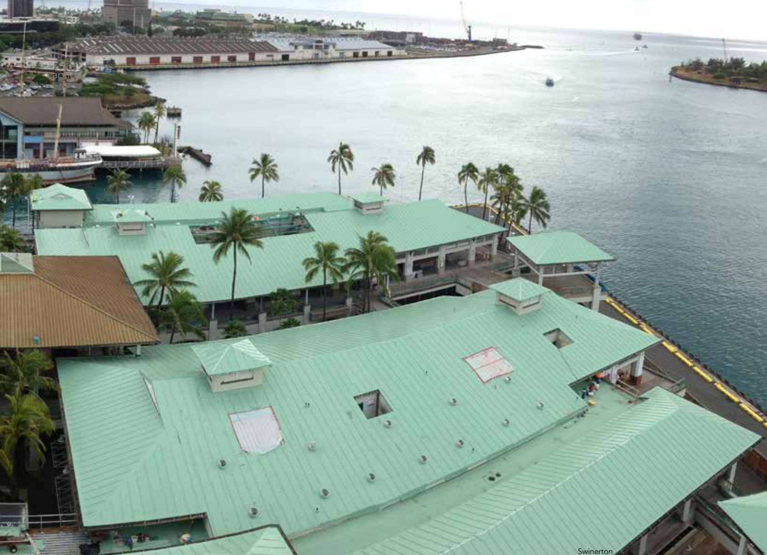
above: A cool view of the complex's new cool roof.
