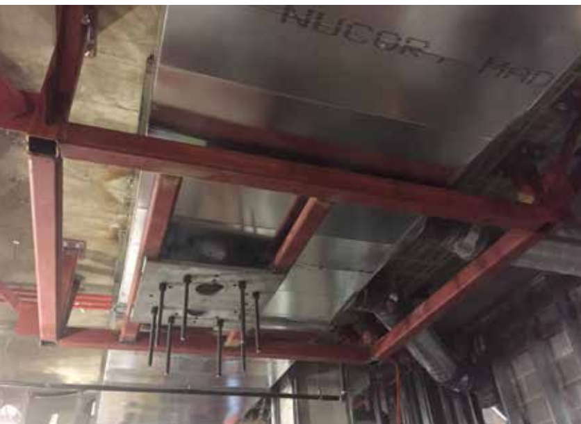
Erection of the connector building steel.
