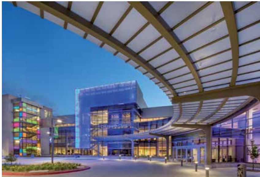
right: The canopy includes six column locations spread along an approximate 52-ft radius.
