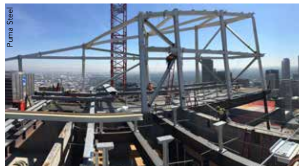
Framing for the crown.
