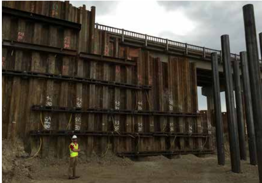
Temporary shoring to support the roadway near the proposed south abutment.
