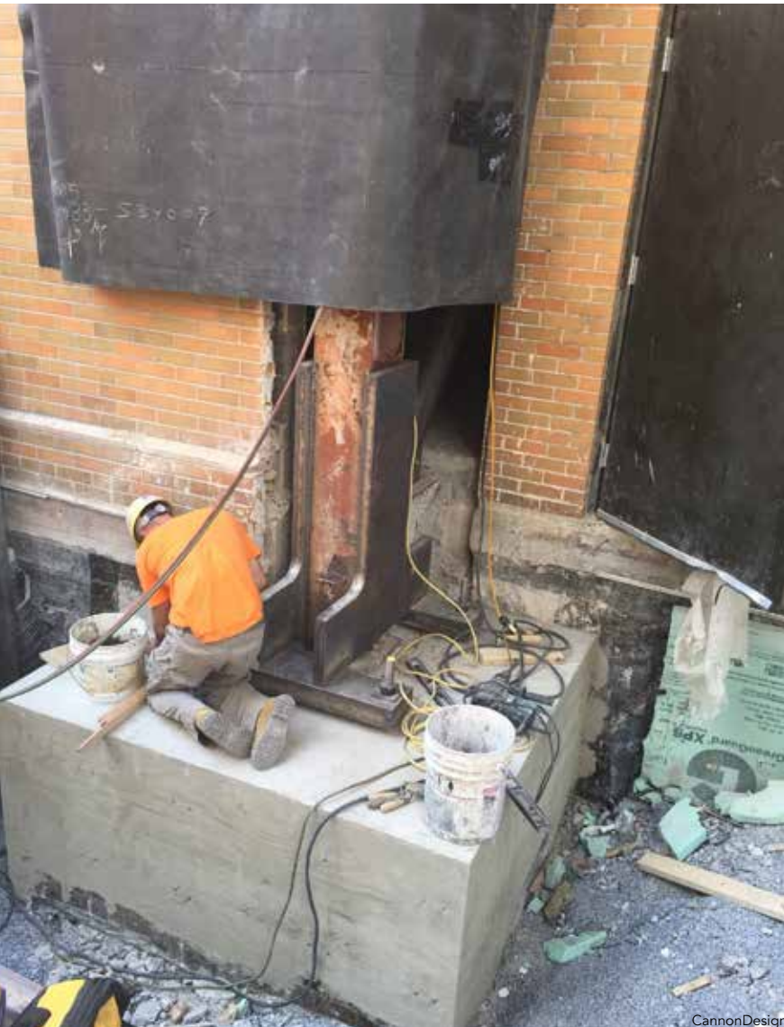
Existing columns required extensive modification to transfer braced frame forces to the foundation.
