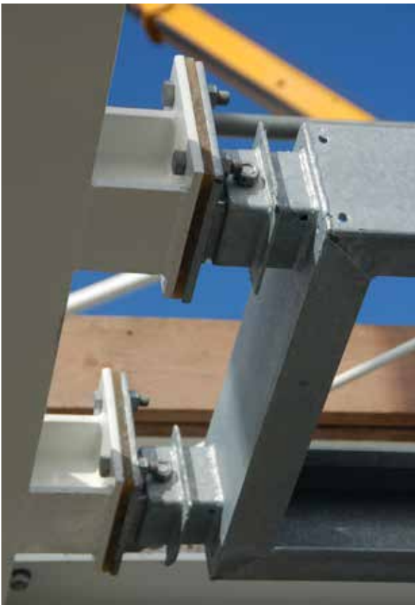
left: Farrat structural thermal break (FSTB) plate. right: A steel-to-steel connection using an FSTB plate.
