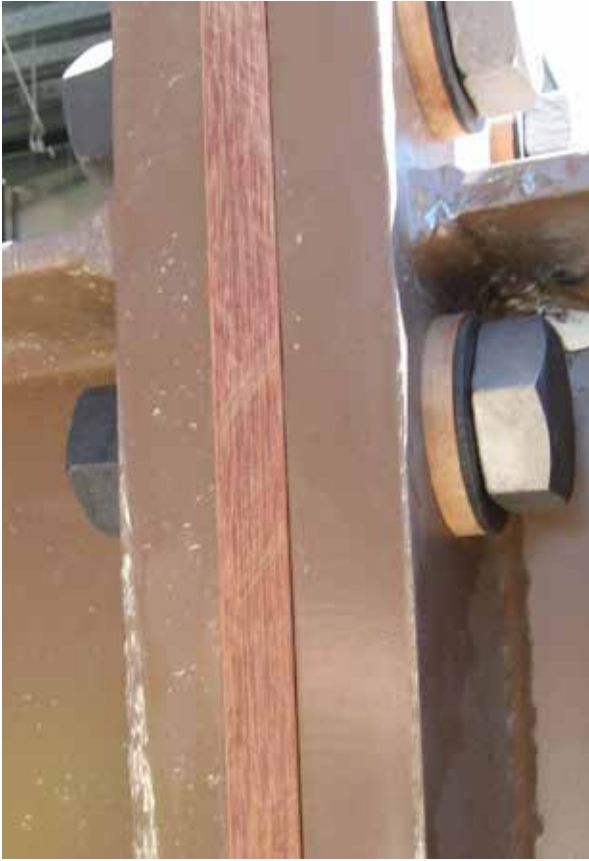
left and right: The Armatherm thermal break system.
