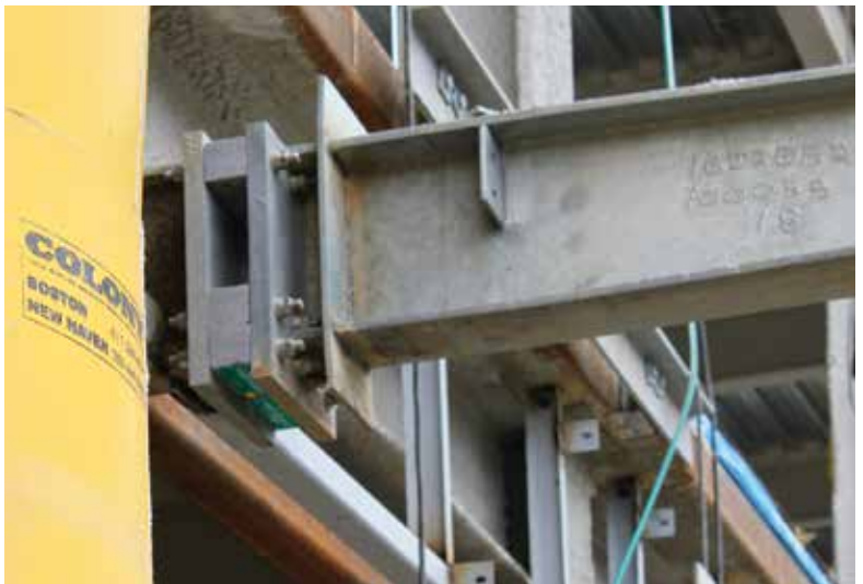
The Life Science Laboratories building at the University of Massachusetts, Amherst (UMass)—fabricated by AISC member and certified fabricator Capco Steel Erection Company—incorporates Schöck’s Type 22 structural thermal break where steel cantilevers penetrate the insulated building envelope, reducing heat loss by approximately 50% at each penetration.
