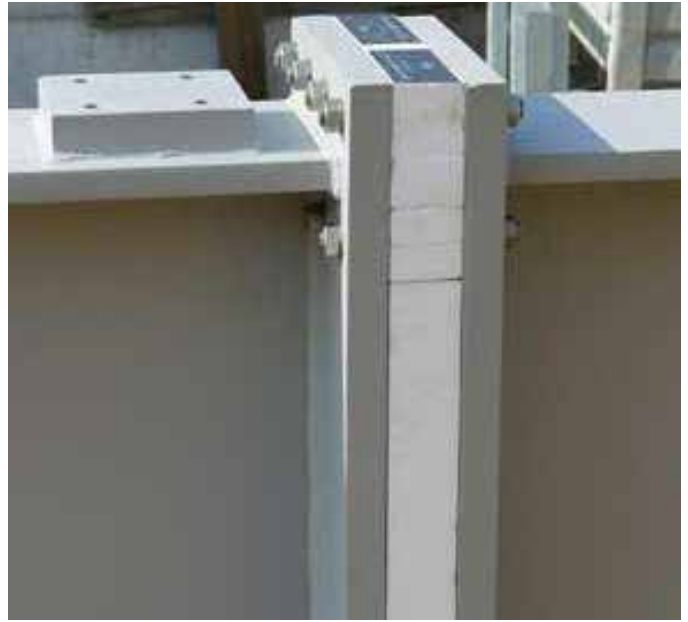
Schöck’s Isokorb thermal break pad between two steel members.
