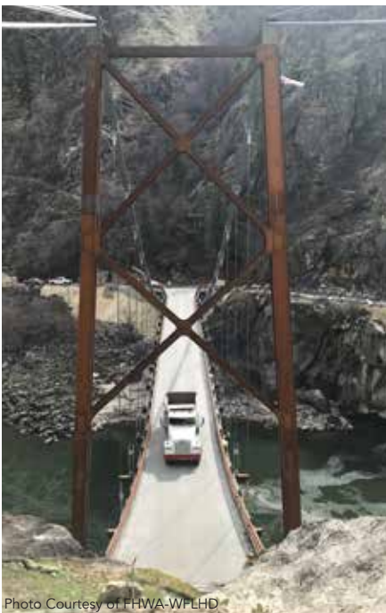
A minimum tower height of at least 60 ft was required in order to place anchorages on favorable rock geometry.
