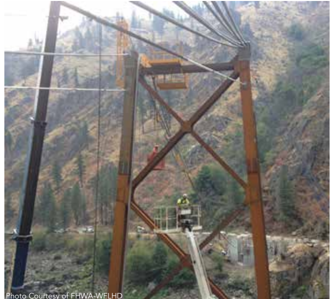
Cable installation from the tower to the south abutment anchorage.
