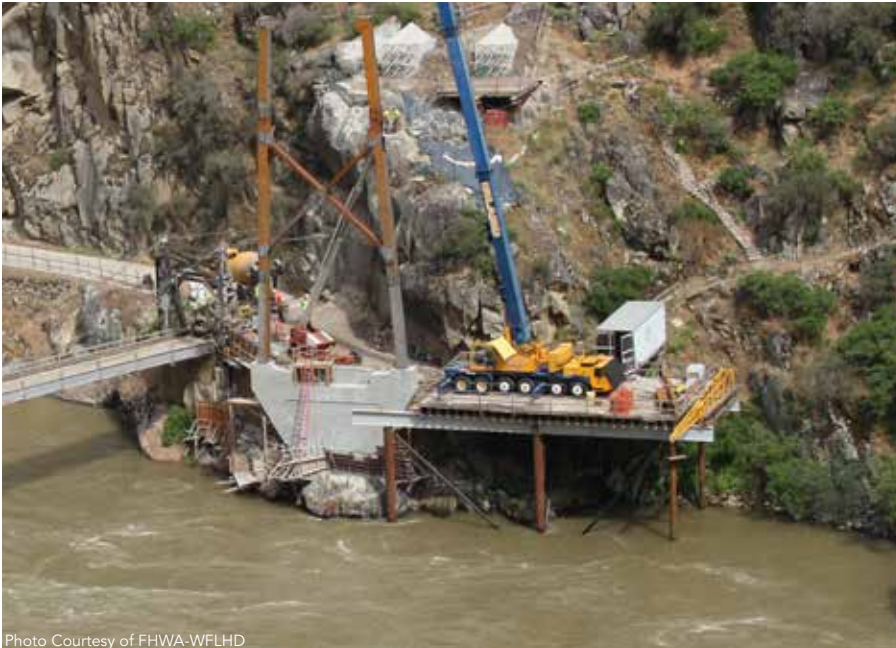
Erecting the tower from a temporary crane platform.
