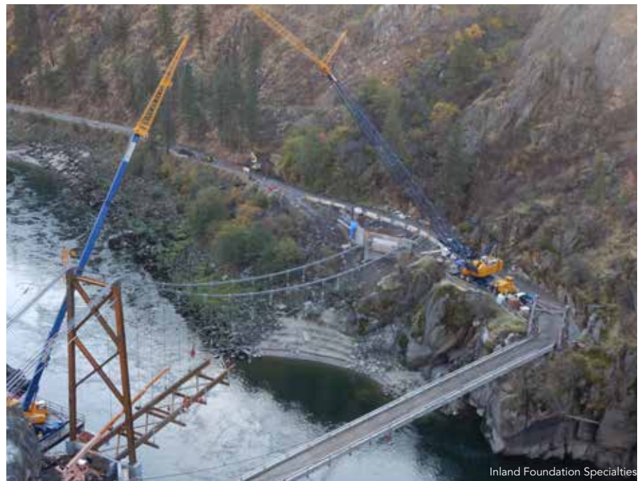
A view of the fixed crane positions for superstructure erection.
