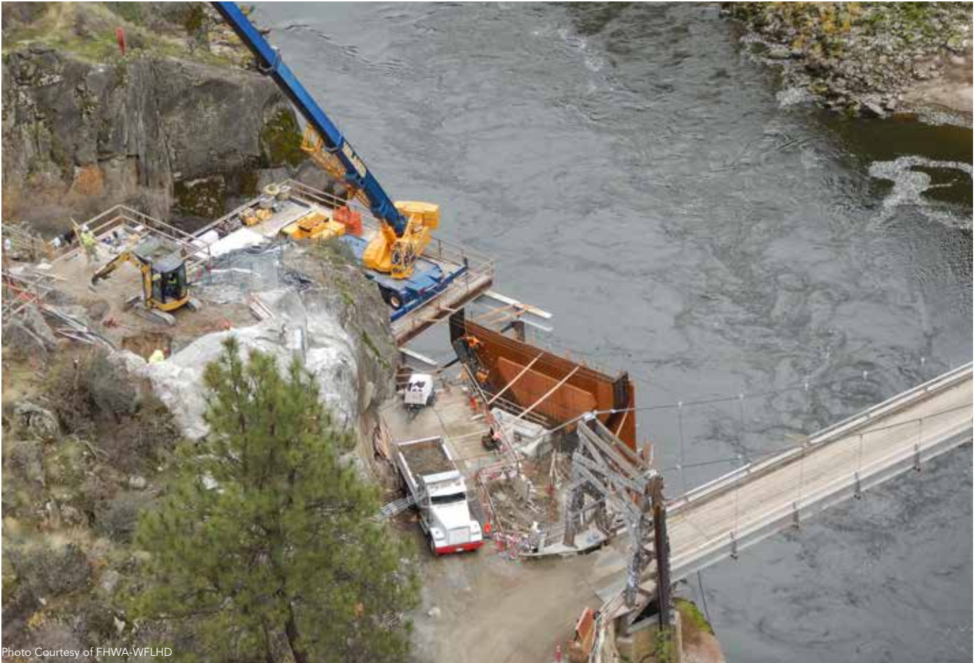
Temporary erection platforms on the north side of the river.
