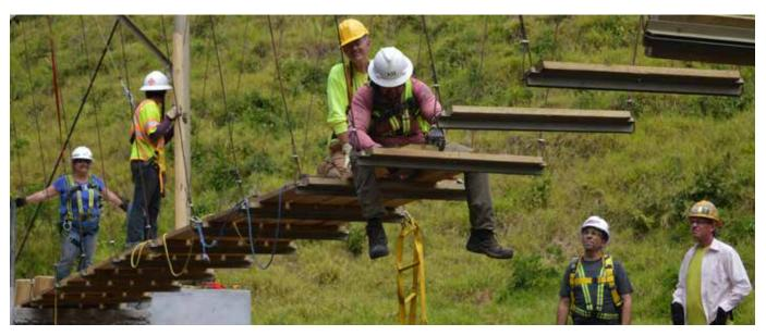
Carter Bearden and Gary Kinchen installing decking near the middle of the bridge span.
