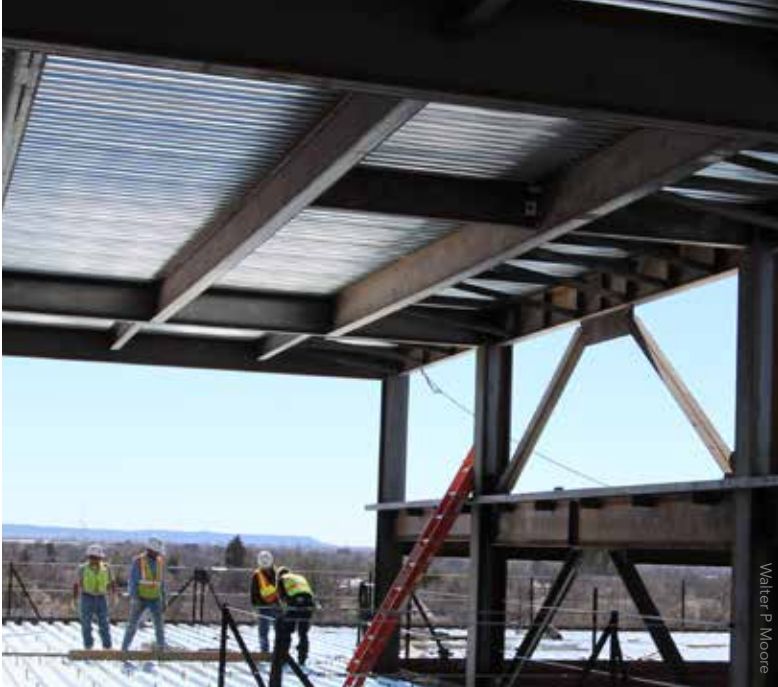
above: Steel bracing at the main roof and high roof.
