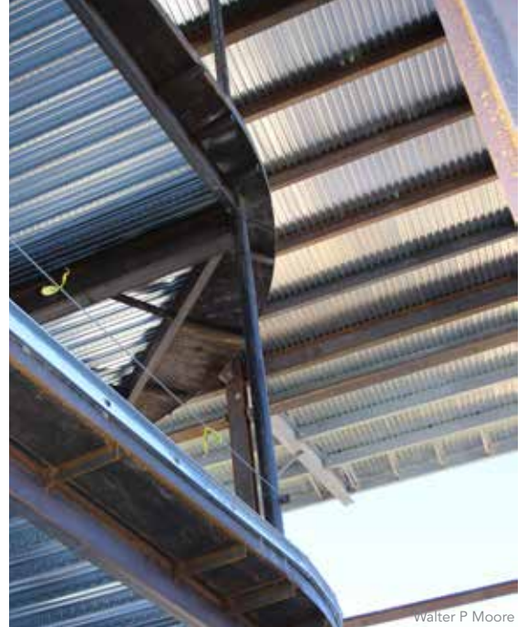
above: Framing for the pod assembly, which hangs from the ceiling in the atrium space.
