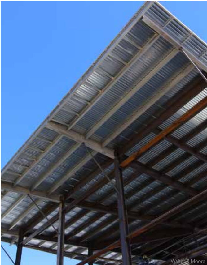
Cantilevered framing for the roof.
