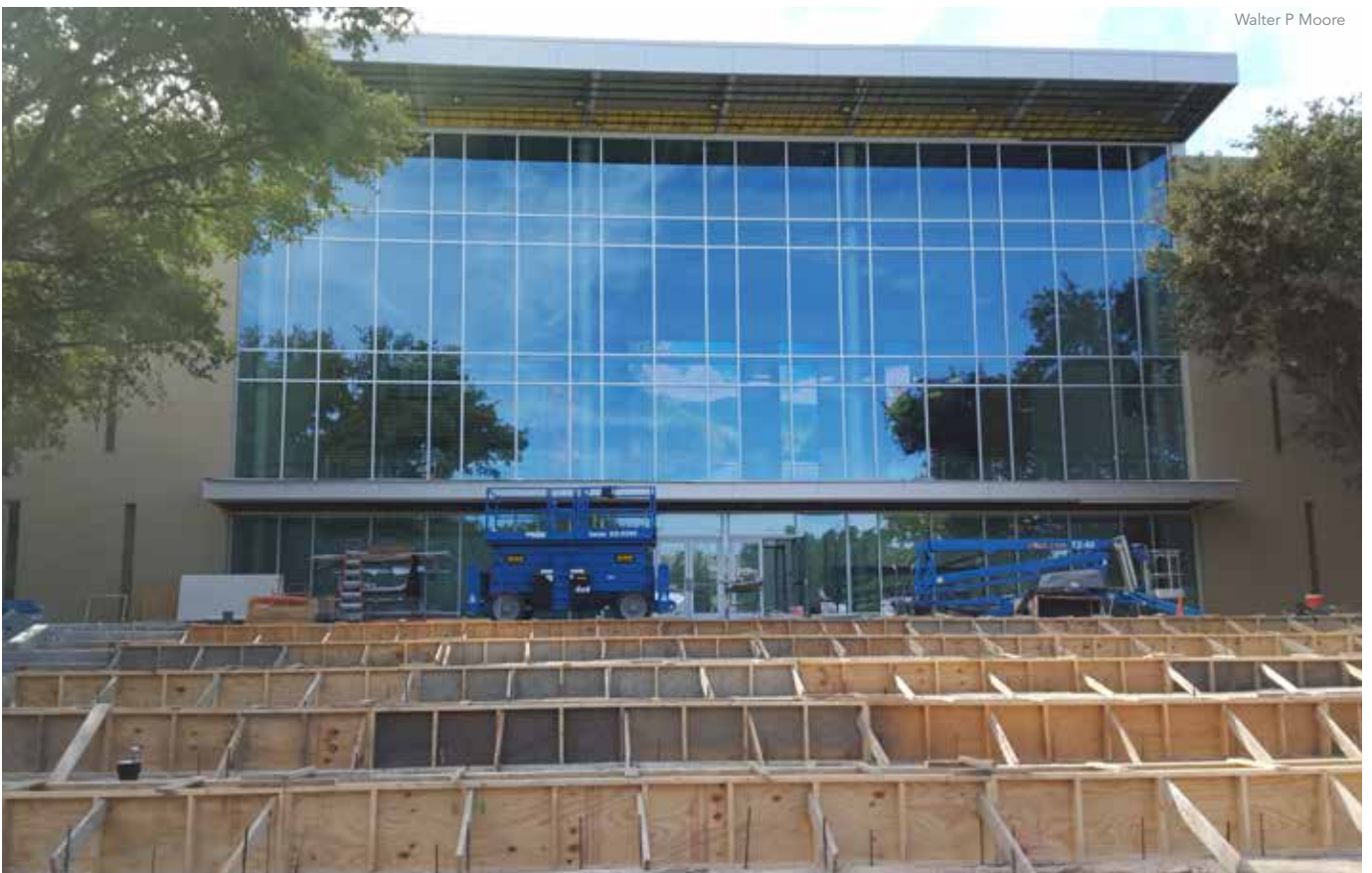
The tall glass façade is uninterrupted by columns and topped by a thin-profile cantilevered high roof.
