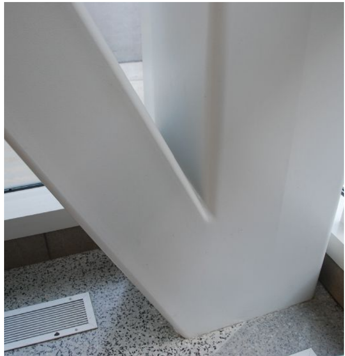
A seamless appearance was essential for the visual success of the connection between these two HSS sections. The result would have been improved had the weld seam on the right-hand section been oriented away from view and towards the window.
