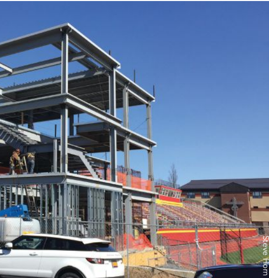
Erecting the stair framing.
