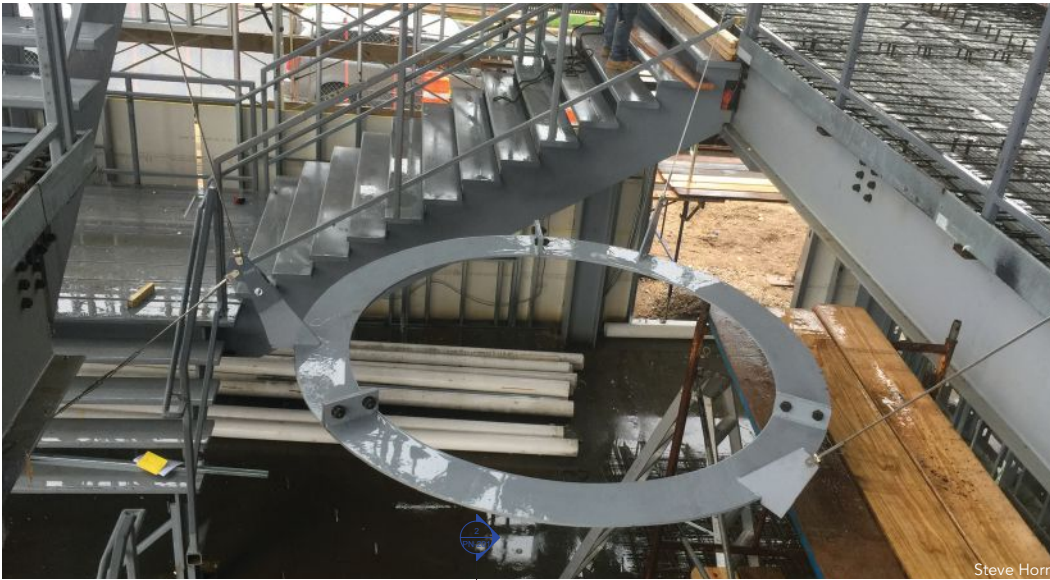
above: Installing the pin ring.
