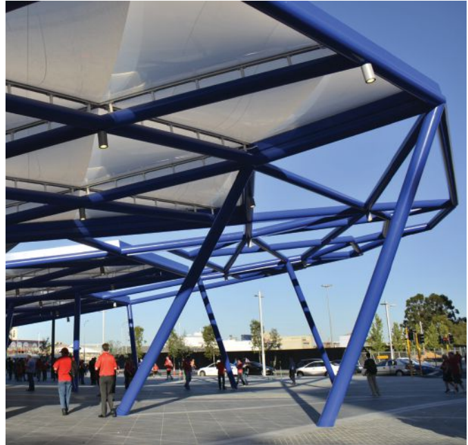
above, right: In order for the HSS-to-HSS connections on this canopy to achieve a precise final appearance, pre-planned weld remediation was necessary. The steel is situated low enough for visual scrutiny.
