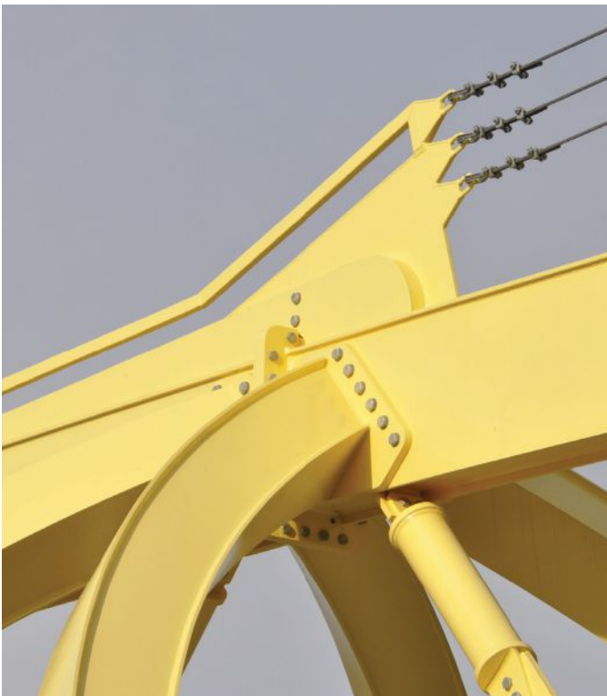
Although this project required significant custom plate work to create its curved box elements, fillet welding was used and weld grinding avoided. The simple inset of the plate provided space for the weld and created an attractive shadow line in the detail.
