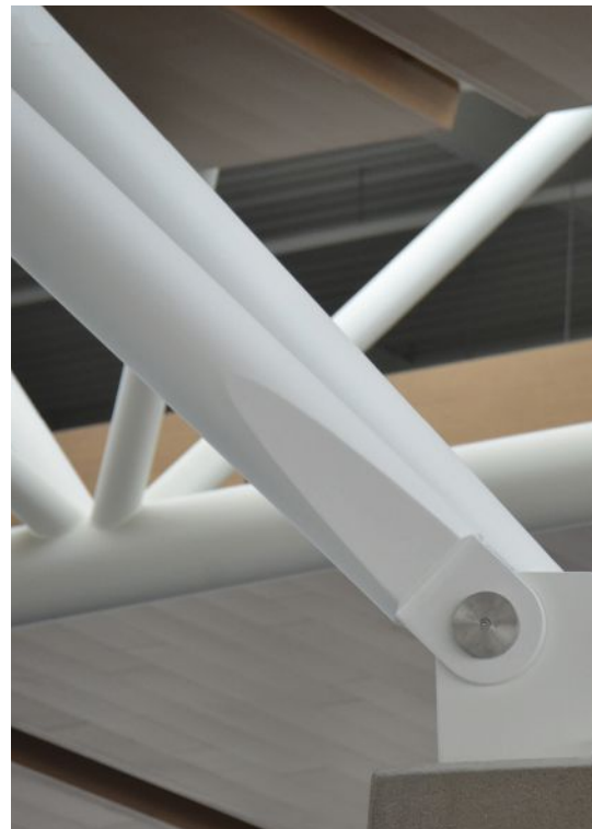
above: Details like as this typical AESS 3 pin connection will always require weld remediation. The parabolic cut in the tube where it is attached to the plate insert will need to be remediated to create a smooth-looking taper.
