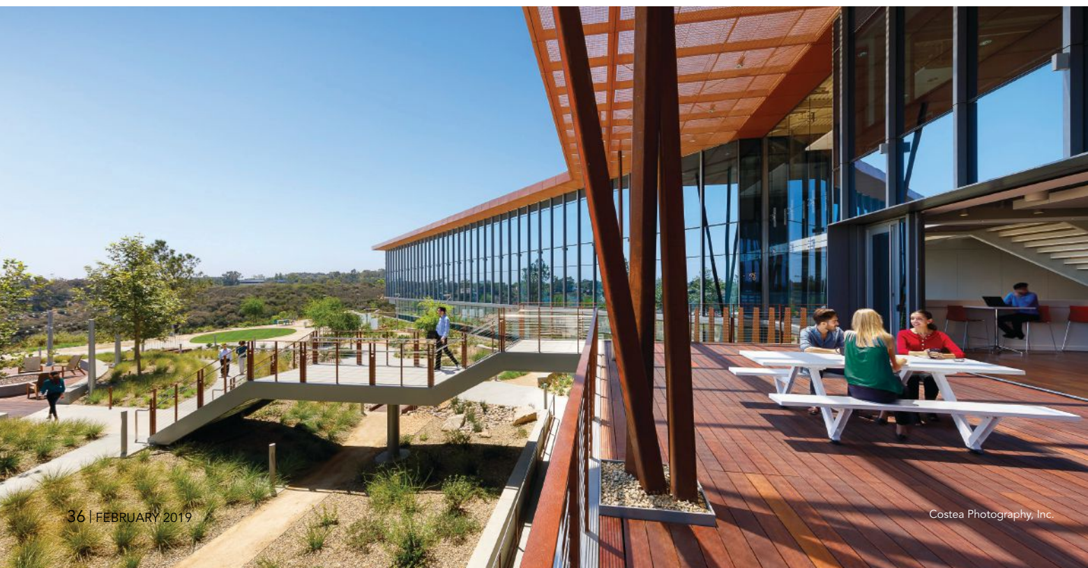
below: The facility consists of 170,000 sq. ft of state-of-the-art laboratory, office and collaboration spaces above two levels of underground parking in the heart of San Diego's Torrey Pines life sciences cluster.
