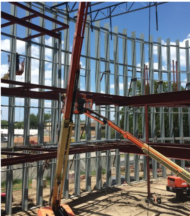
below: The fins were installed in 10-ft-wide modules.
