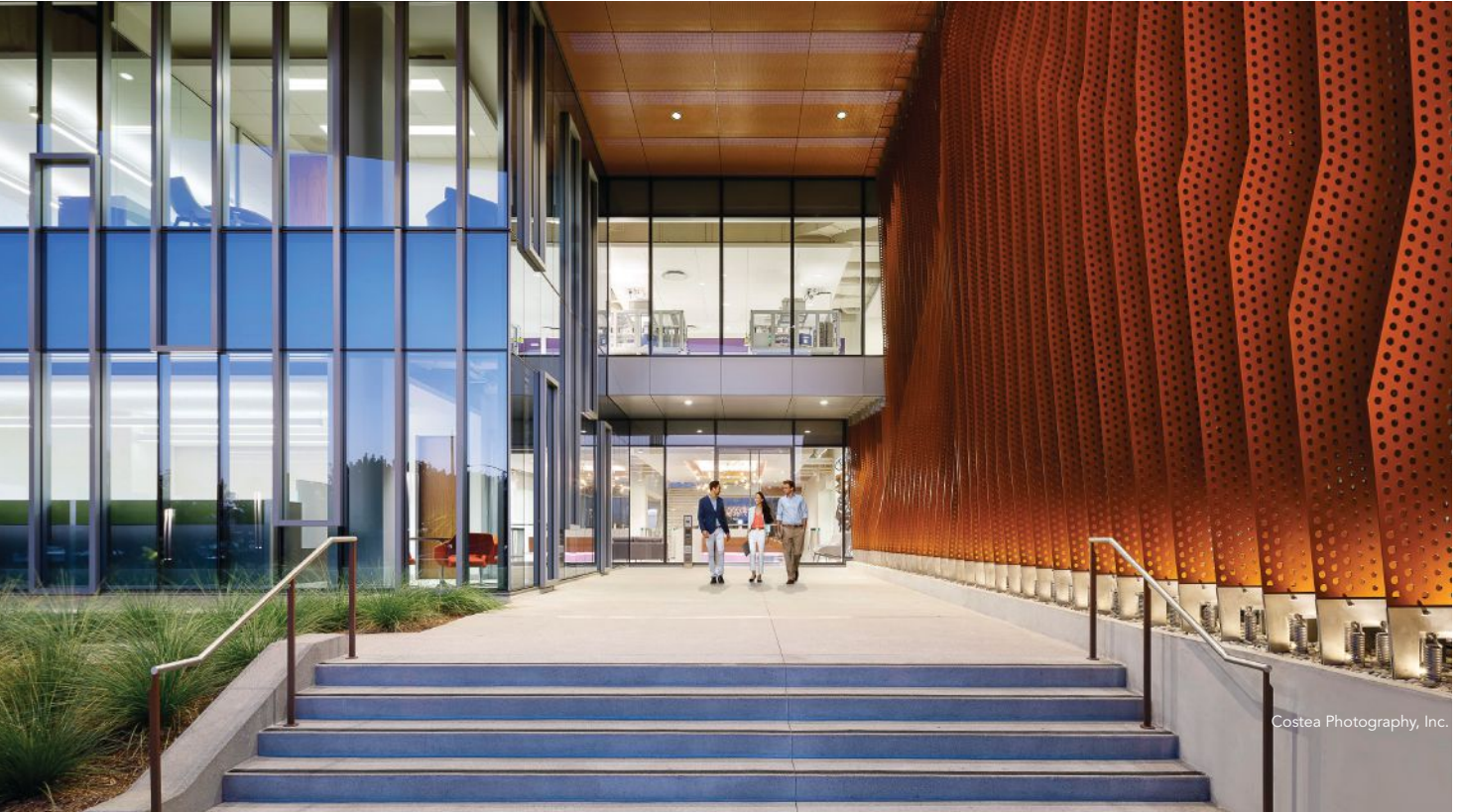
The design team chose a stepped-grade, steel-framed concept for the building, comprised of two rectangular wings interconnected by a high-volume through lobby.
