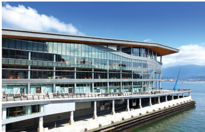
VANCOUVER CONVENTION CENTER EXPANSION PROJECT
