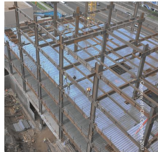
The new tower adds one below-grade and six above-grade levels and was designed with the option to expand vertically by three floors.
