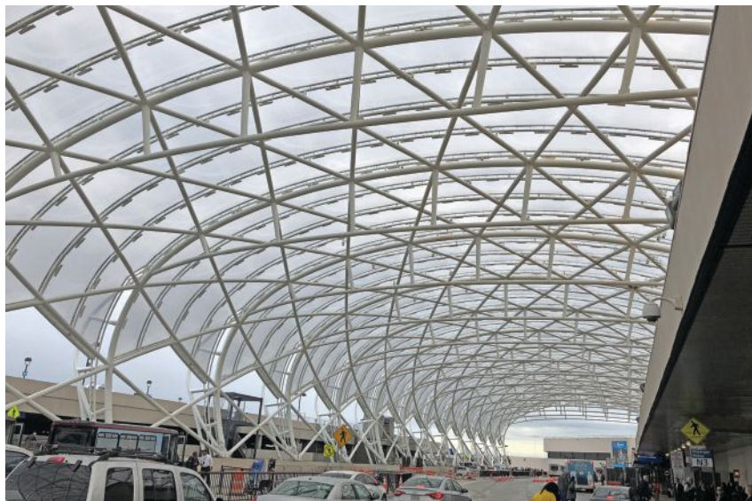
below: The new curved canopy at Hartsfield-Jackson Atlanta International Airport.
