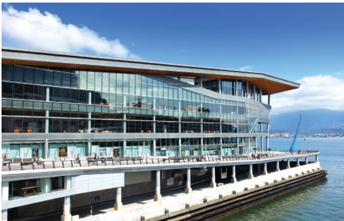
VANCOUVER CONVENTION CENTER EXPANSION PROJECT
