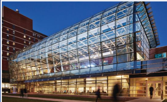
2014 SEAIO Best Project - Elliptically curved trusses rolled from 5" and 8" diameter AESS pipe for Institute of Environmental Sustainability at Loyola University. Chicago, IL
