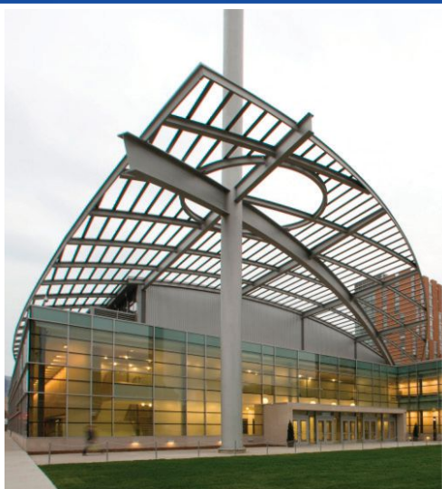
2010 NCSEA Award Winner - 200 tons of beams, channels and angle for the roof of the University of Illinois at Chicago Forum. Chicago, IL
