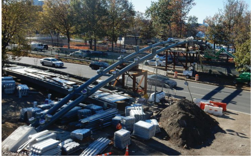
above and below: Erecting the bridge over Storror Drive.
