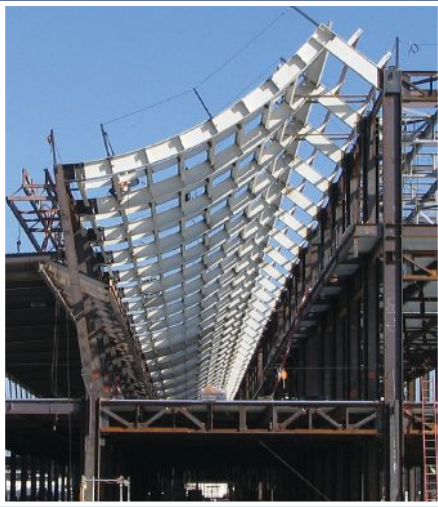
2011 IDEAS 2 National Winner - 420 tons of rectangular tubing, pipe and beams for the roof at the Norman Y. Mineta San Jose International Airport. San Jose, CA
