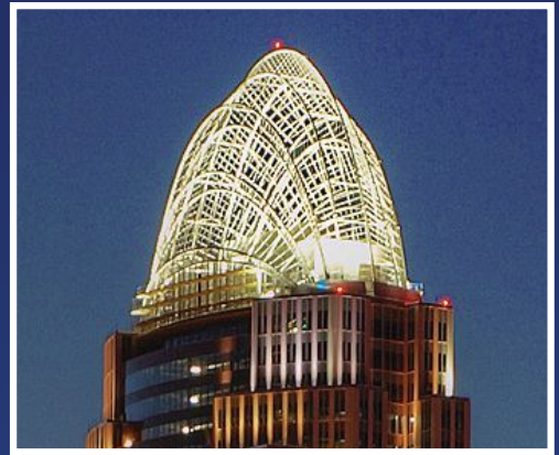
2012 IDEAS 2 Merit Award - 133 tons of 16" pipe curved for the Rooftop Tiara of the Great American Tower at Queen City Square. Cincinnati, OH
