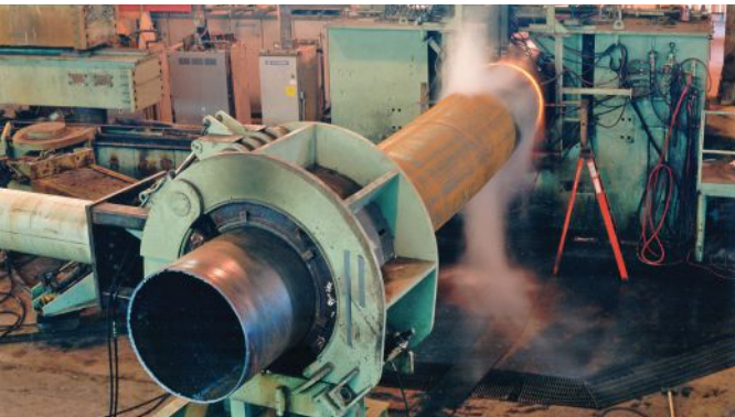
below: Heat induction bending.
