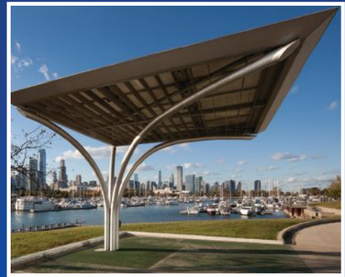
2013 IDEAS 2 Merit Award - 3600 pounds of pipe each curved with multiple radii for a solar canopy to recharge batteries on electrical vehicles. Chicago, IL
