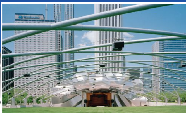
2005 EAE Merit Award - 570 tons of 12", 14", 16", 18" and 20" pipe curved for the Jay Pritzker Pavilion. Chicago, IL
