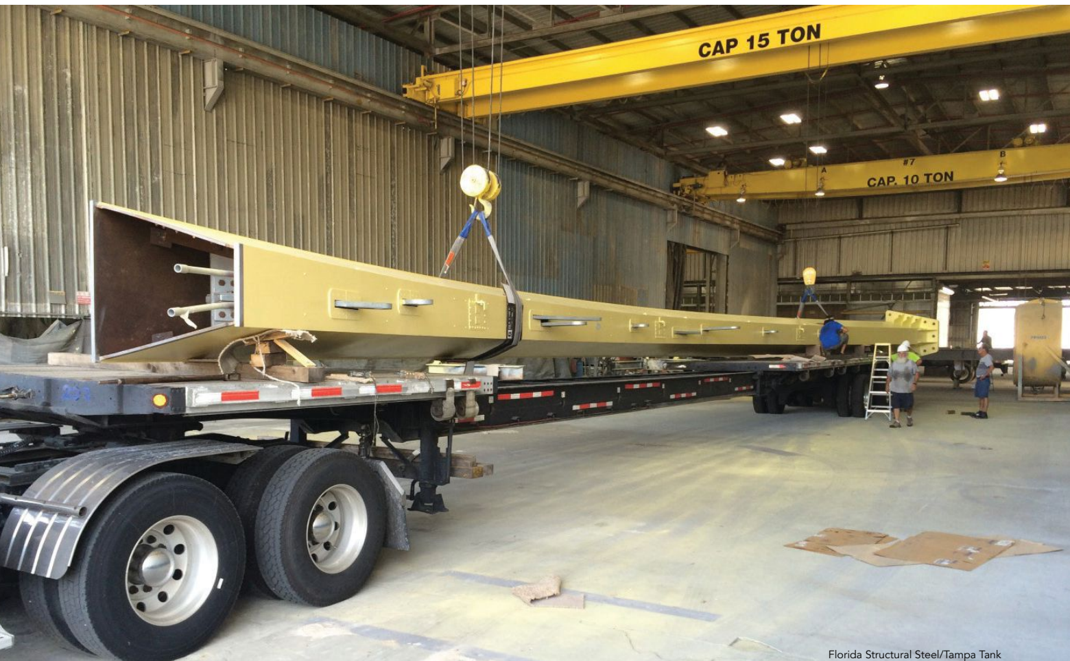
above: Shipping a completed half of an arch-rib girder from the fabrication facility. below: The pedestrian and vehicle bridge carries 2nd Street over Austin's Shoal Creek.
