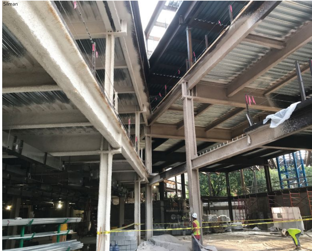
An intersection of the steel framing for multiple bars.
