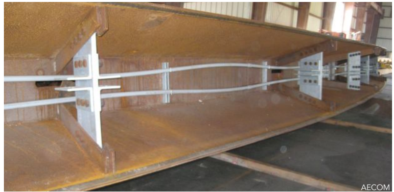
An inside look at one of the bridge's arch ribs during fabrication.
