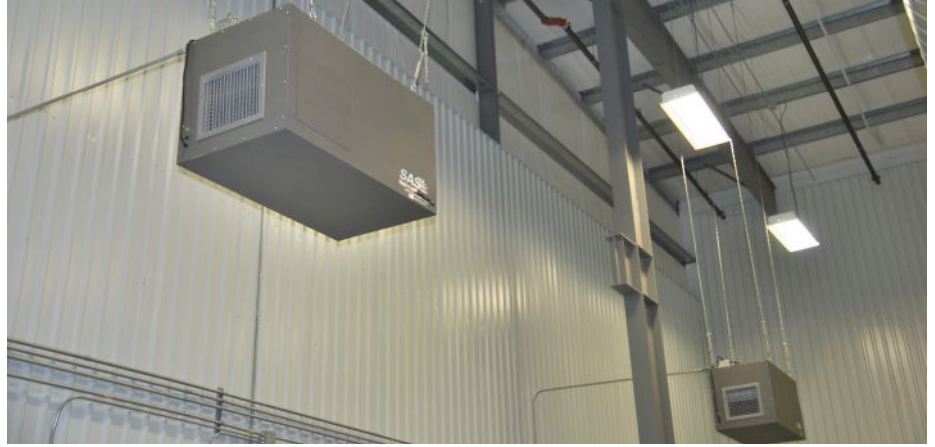
Hanging ambient air cleaners, such as the models seen here, are advised to be used with a source-capture fume extractor.
