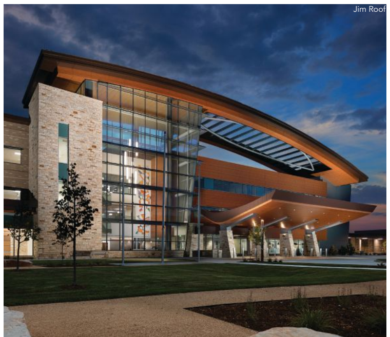
below: The “scoop” design of the ground-level entry canopy was designed to complement the exposed arch roof.
