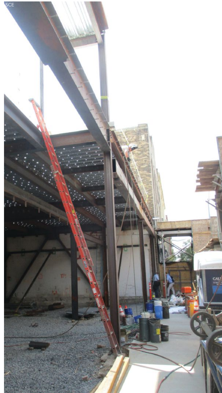
above: The roof structure was made up of new W14×34 ASTM A992 members supporting a new \frac{3}{4} -in. lightweight concrete slab on 2-in.-deep galvanized composite metal deck.
