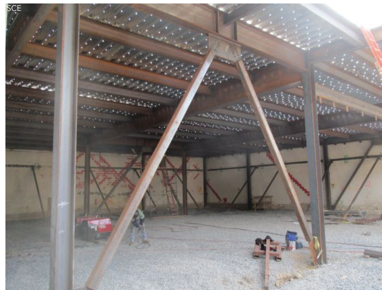
above and left: The braces are supported by a spread footing system, above which concrete piers connect to the columns of each chevron brace.
