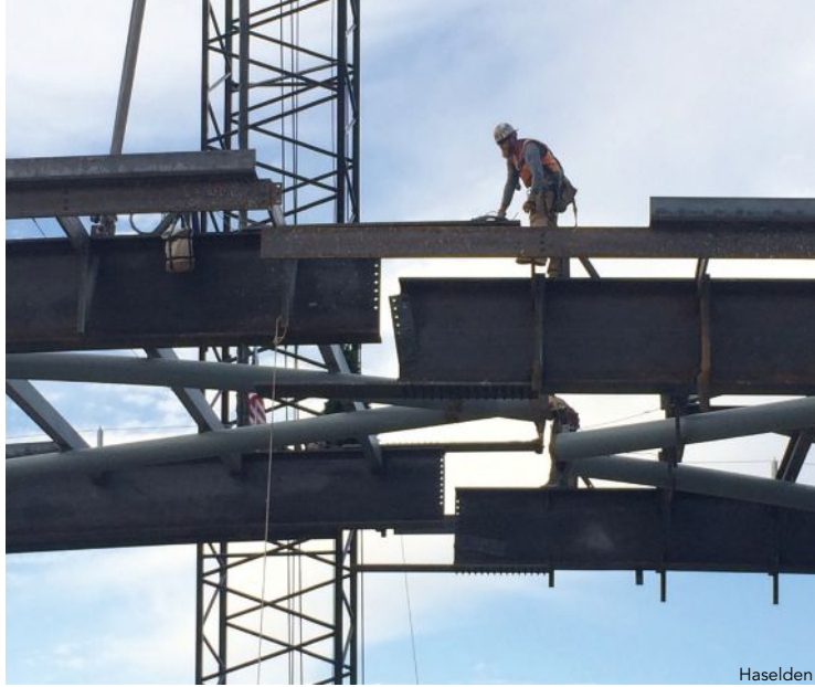
Connecting the 150-ft clear-span segment with the lobby roof segment via bolted splices.
