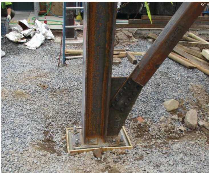
above and left: The braces are supported by a spread footing system, above which concrete piers connect to the columns of each chevron brace.
