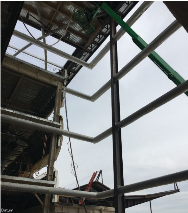
above and below: The exposed steel elements in the lobby were designated as AESS Category 3, as they are within 10 ft to 20 ft from view.
