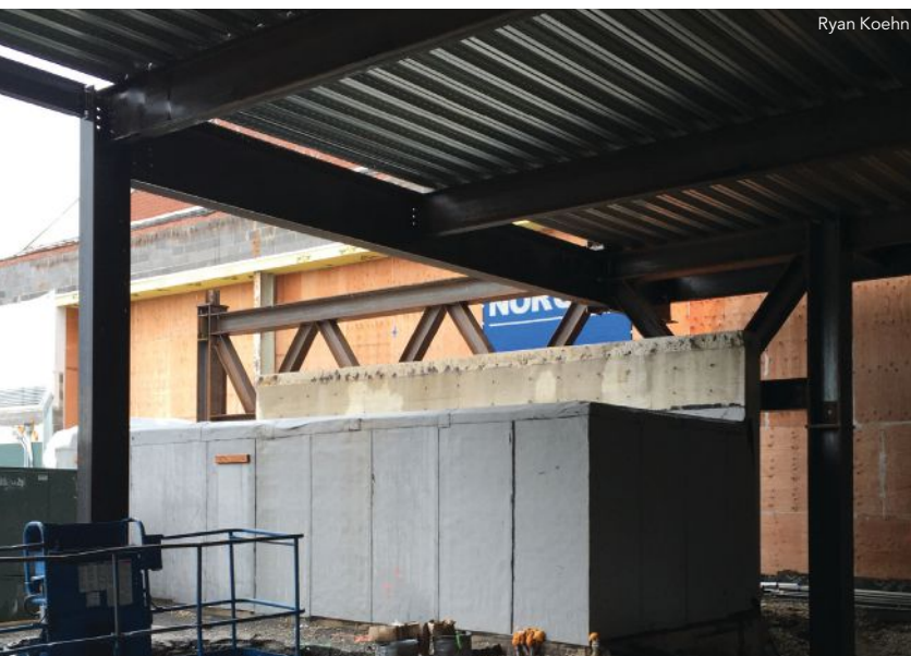
below: A 7-ft-deep truss transfers the upper building levels above an existing high-voltage room at ground level.
