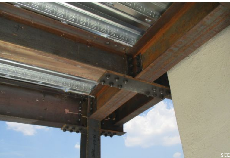
above: The roof structure was made up of new W14×34 ASTM A992 members supporting a new \frac{3}{4} -in. lightweight concrete slab on 2-in.-deep galvanized composite metal deck.
