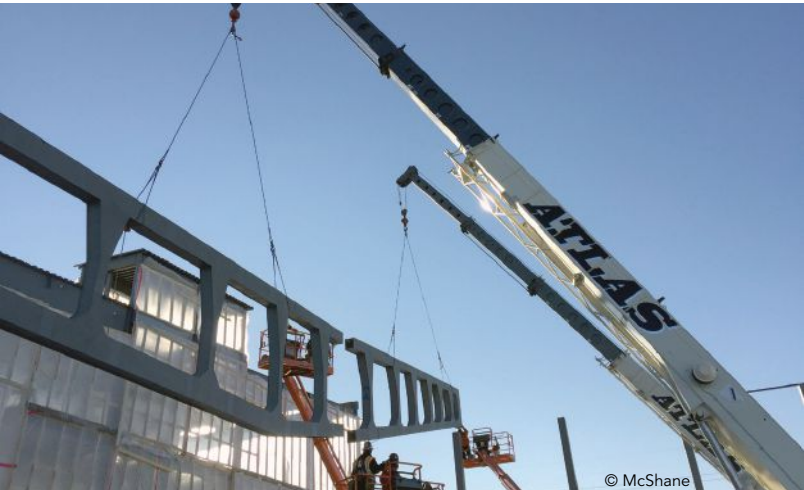
above: The truss erection sequence was as follows: The first two (of three) sections were bolted together on the ground and then picked up with two cranes. After the north end of the truss assembly was attached to the column, the north crane moved to the south end and picked up the south (third) section of the truss and lifted it in place.
