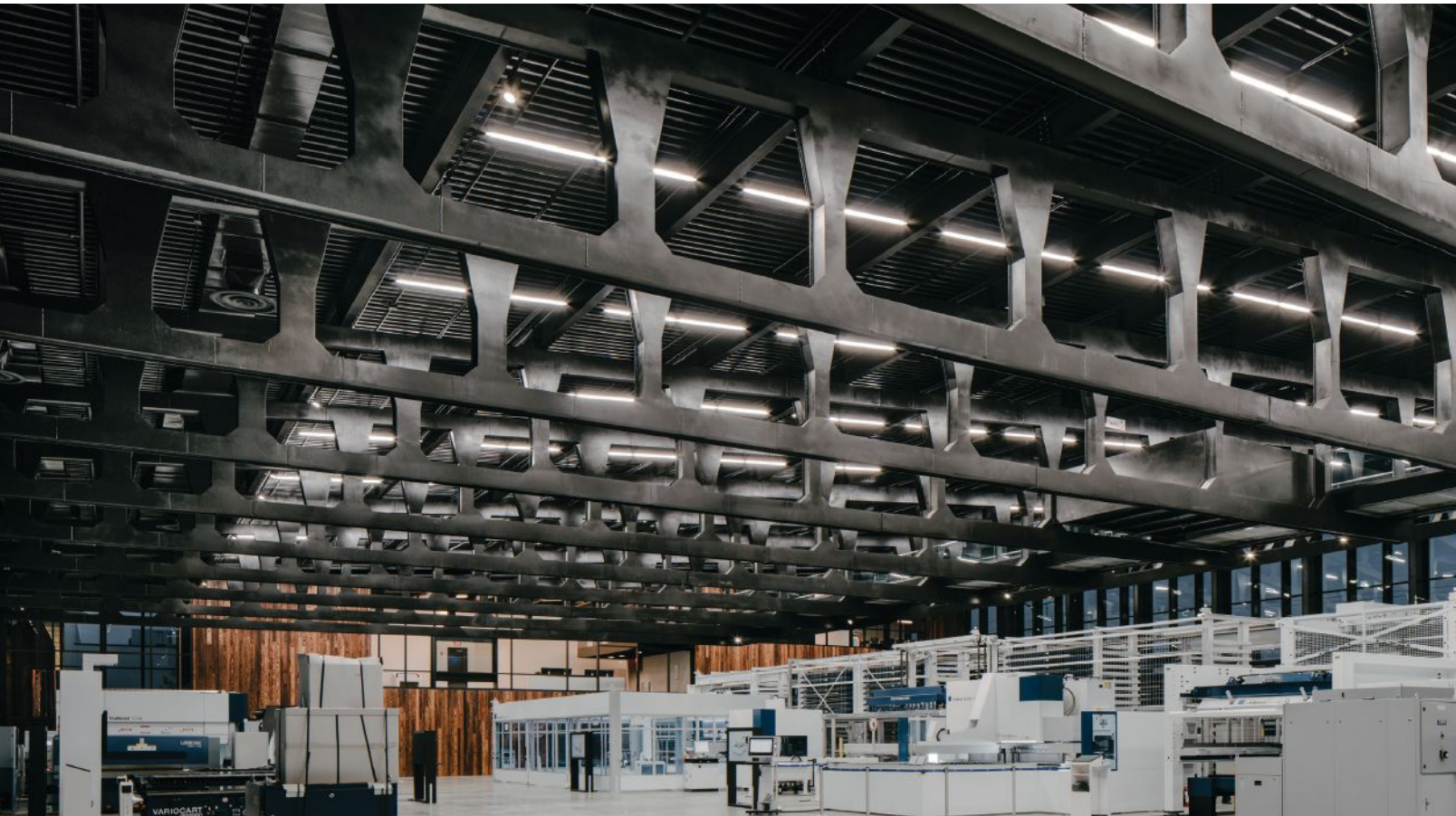
above: The truss erection sequence was as follows: The first two (of three) sections were bolted together on the ground and then picked up with two cranes. After the north end of the truss assembly was attached to the column, the north crane moved to the south end and picked up the south (third) section of the truss and lifted it in place.
