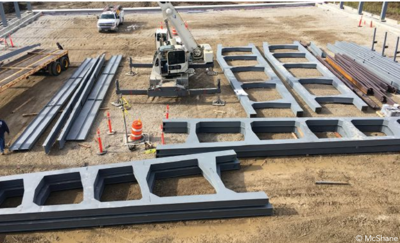
above: The truss erection sequence was as follows: The first two (of three) sections were bolted together on the ground and then picked up with two cranes. After the north end of the truss assembly was attached to the column, the north crane moved to the south end and picked up the south (third) section of the truss and lifted it in place.
