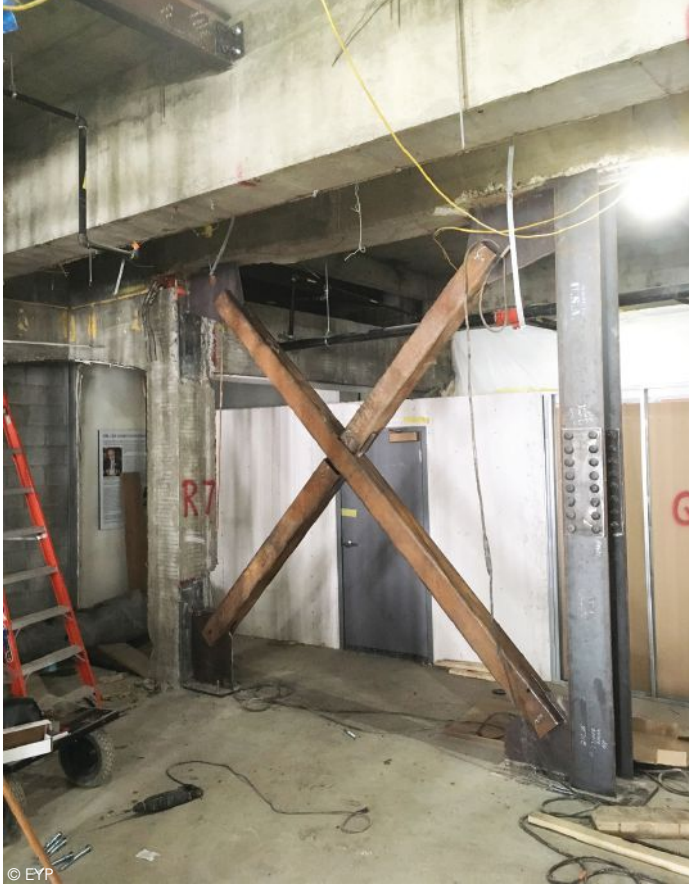
One of eight braced frames installed throughout the existing building. The left column is part of the original construction, and the right one is new.
