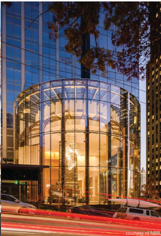
The Great Room is a 45-ft-tall steel-framed entryway rotunda featuring a circular staircase and large glass plates suspended by cables.
