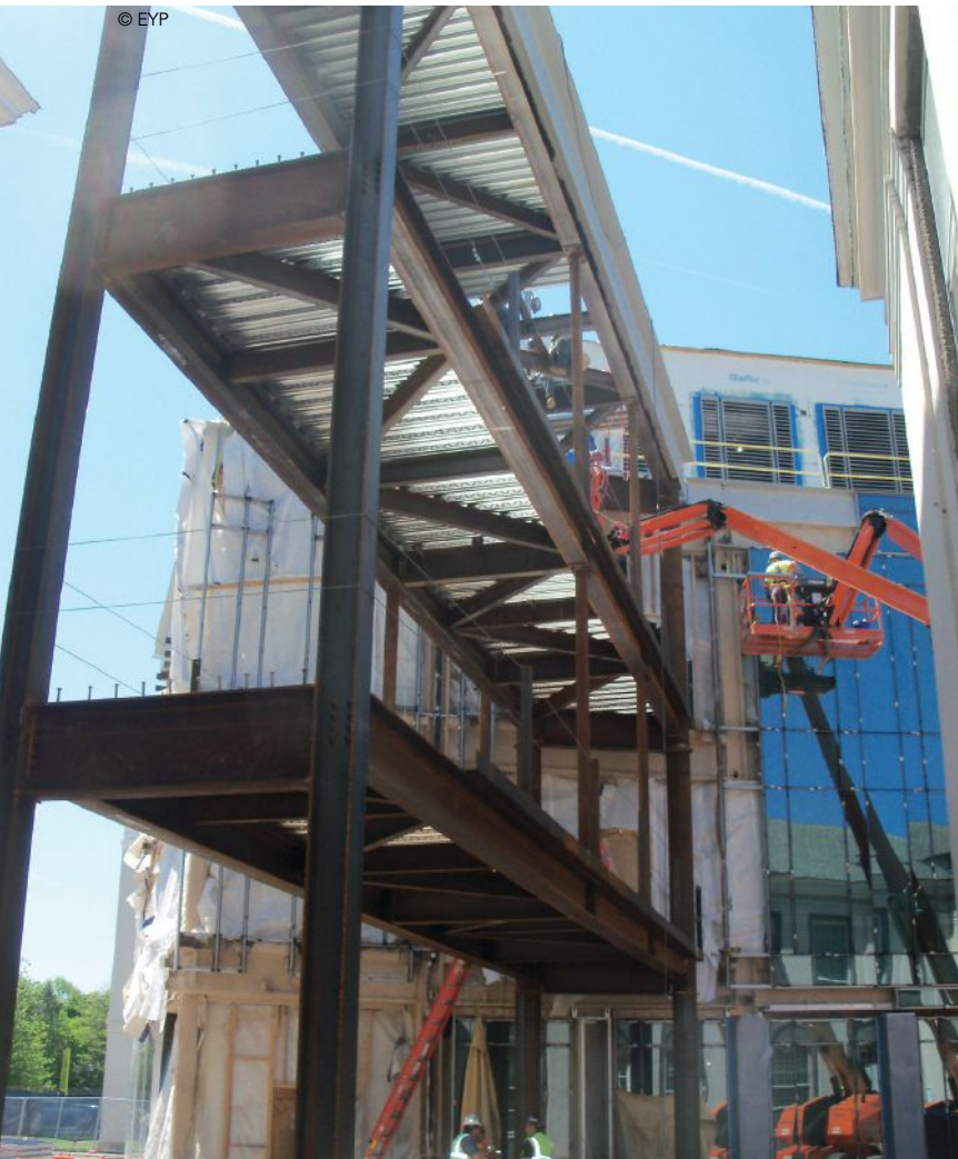
below: The steel-framed, multi-level North Connector joins Steinmetz and Butterfield Halls with Ainlay Hall.
