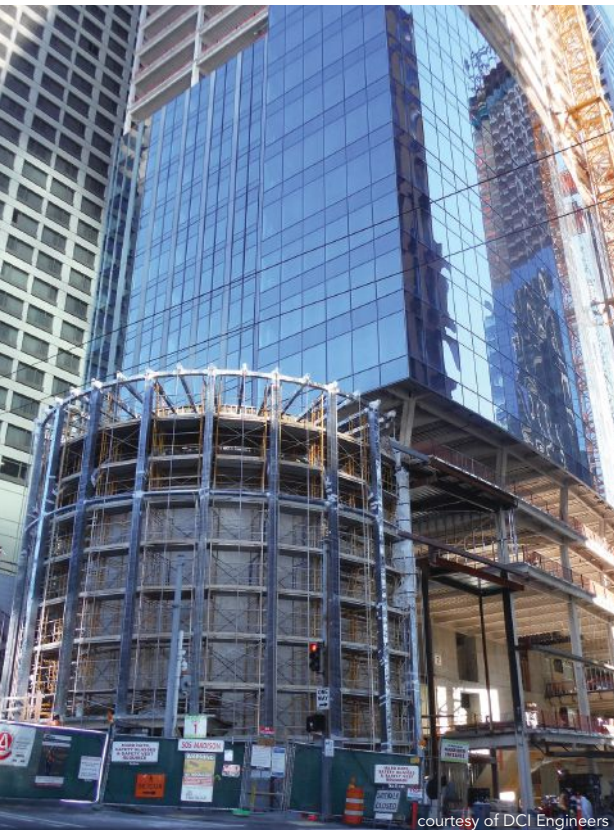
The Great Room is a 45-ft-tall steel-framed entryway rotunda featuring a circular staircase and large glass plates suspended by cables.
