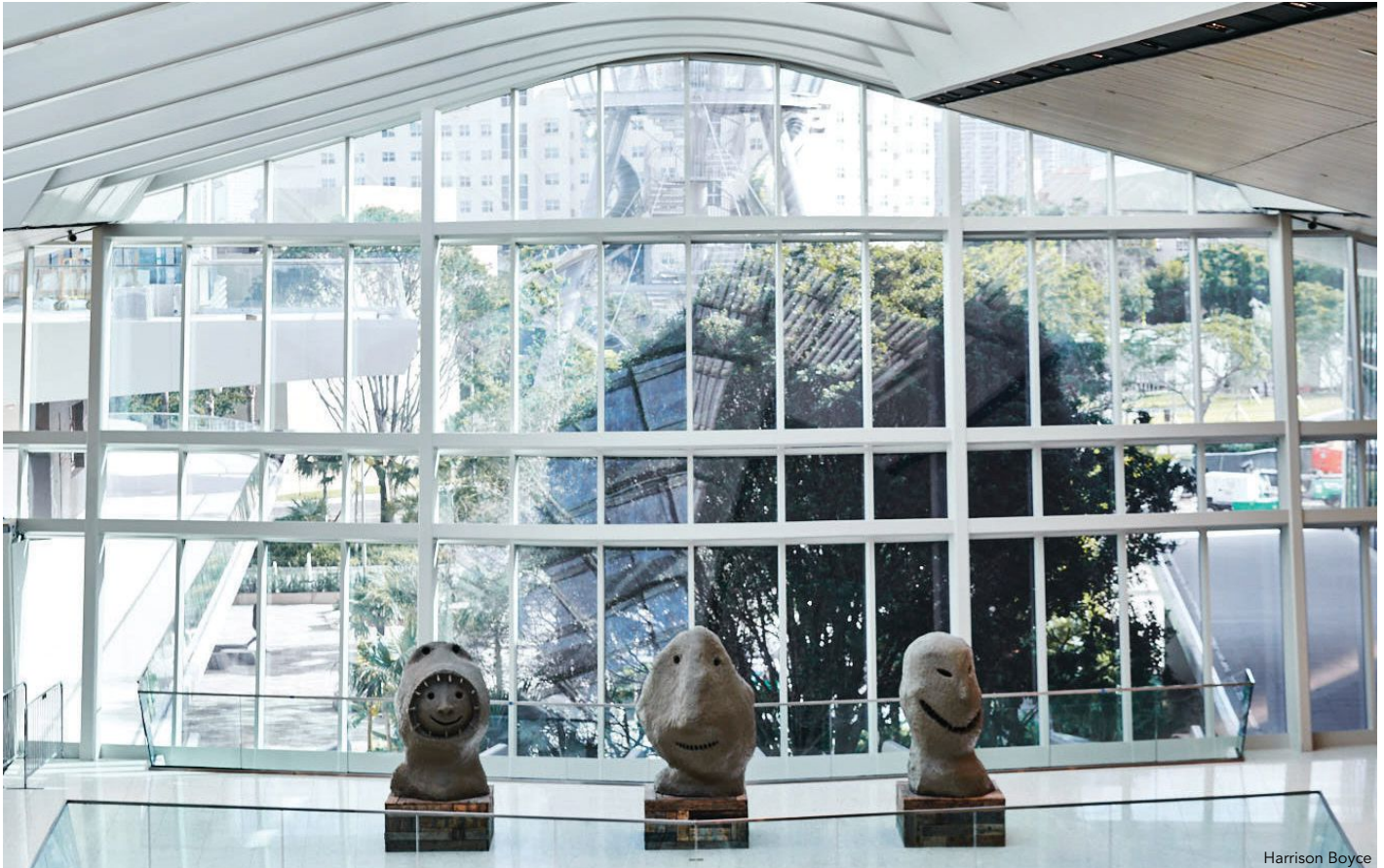
A 51-ft-tall by 80-ft-wide glass wall, supported by steel framing designated as AESS, encloses the northeast end of the concourse. Built-up beams using individual plates form the roof elements.
