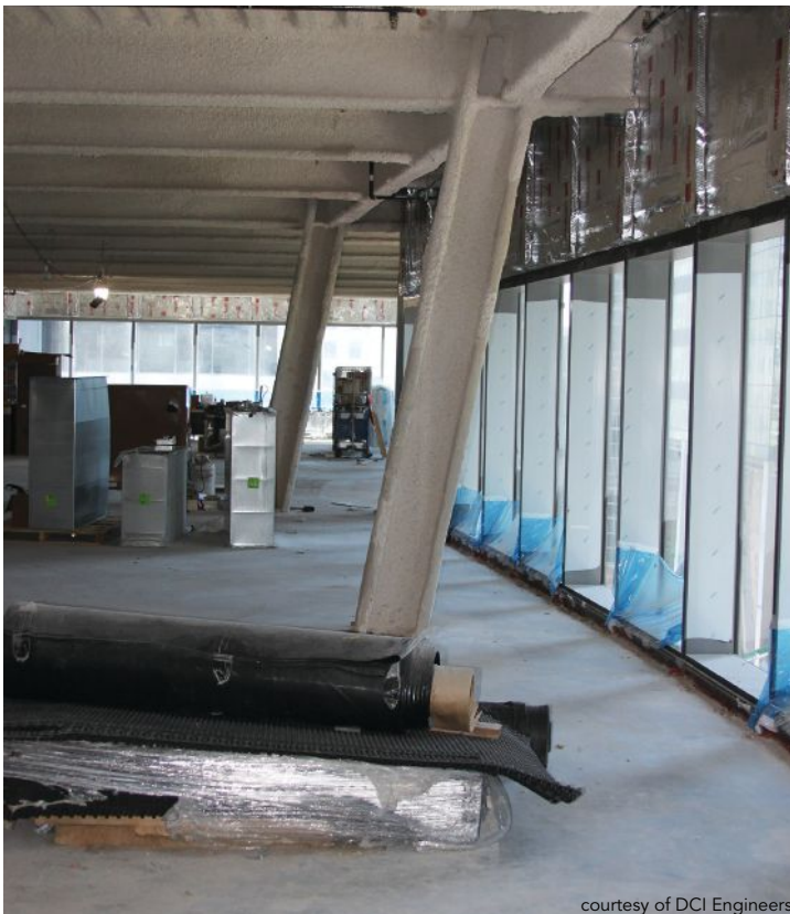
The perimeter tower columns slope outward from Level 3 to Level 6 on two sides of the building.
