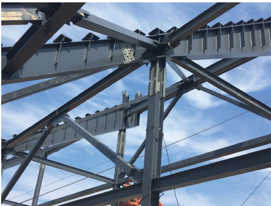
above: Canopy framing and plate girders for the east seating bowl. Column locations above the raised concourse were governed by inflexible seating configurations, so built-up plate transfer girders were used above the easements.
