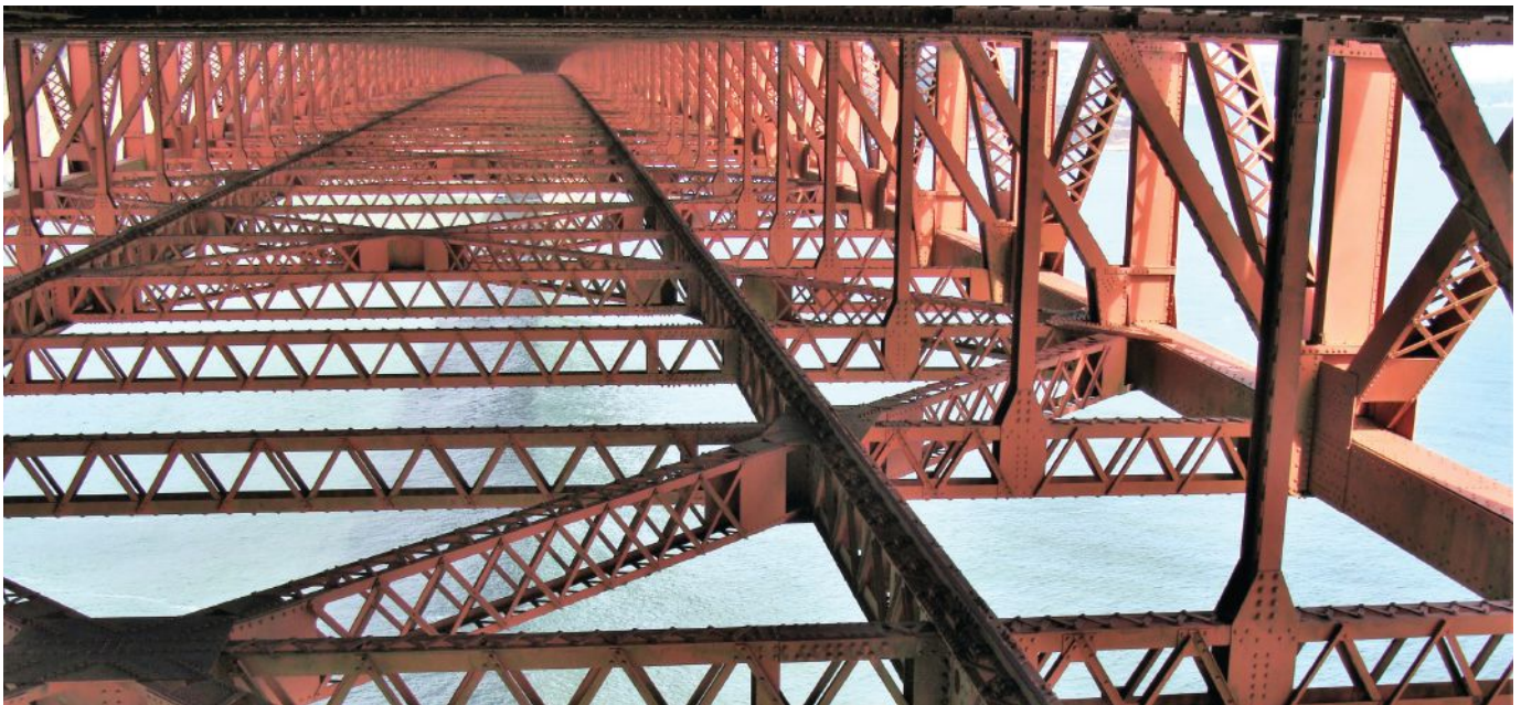
below: The built-up riveted floor truss of the Golden Gate Bridge in San Francisco.
