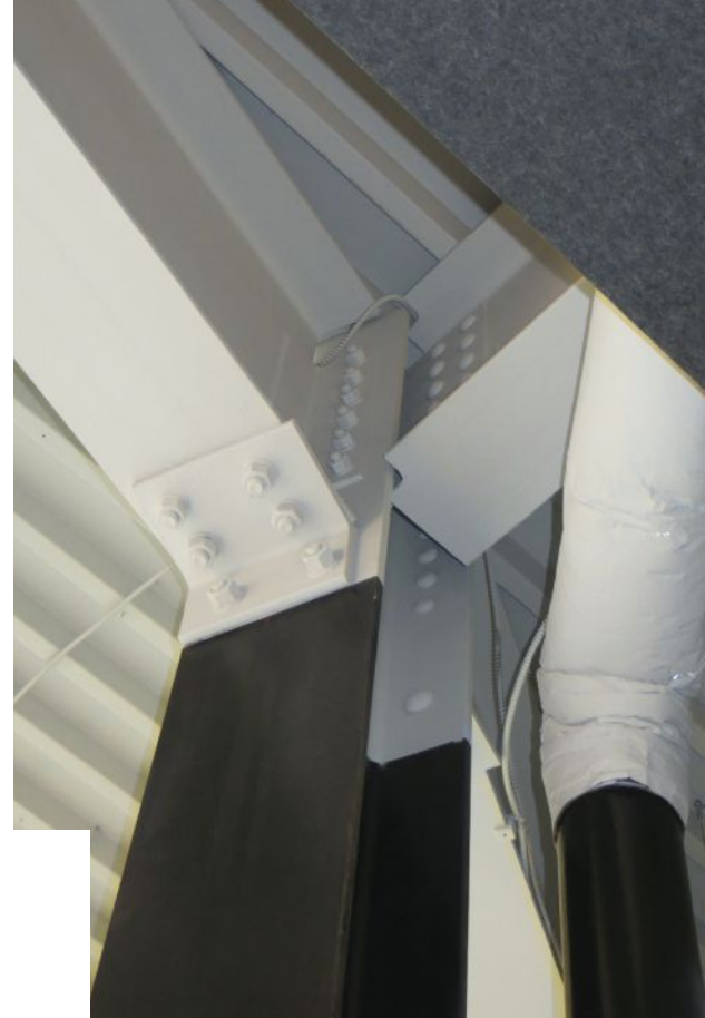
above and left: During the shop drawing phase, discussion between the engineer and fabricator resulted in the development of multiple variations of a partially restrained moment connection to improve constructability.
