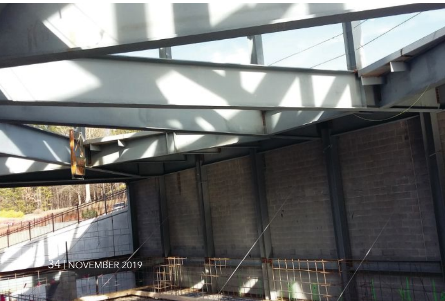
right and below: A radial scheme was used for the W36 transfer beams extending through the middle of the two-story pool area. This design accomplishes the open aesthetic desired by the architect, with natural light from the windows shining through the spaces between the transfer beams and into the pool area.
