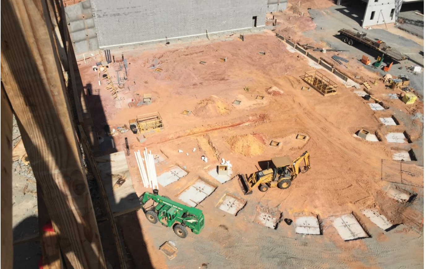
The building's foundations, with the CMU and tie-back wall at top of photo.
