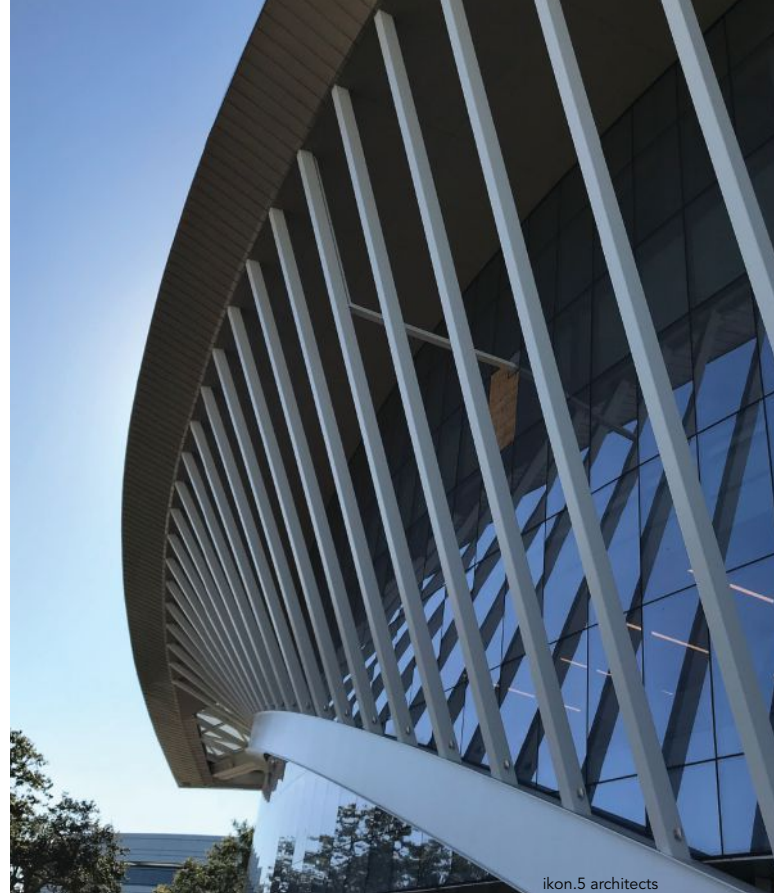
above: A view from ground level showing an exterior arch and struts during construction.
