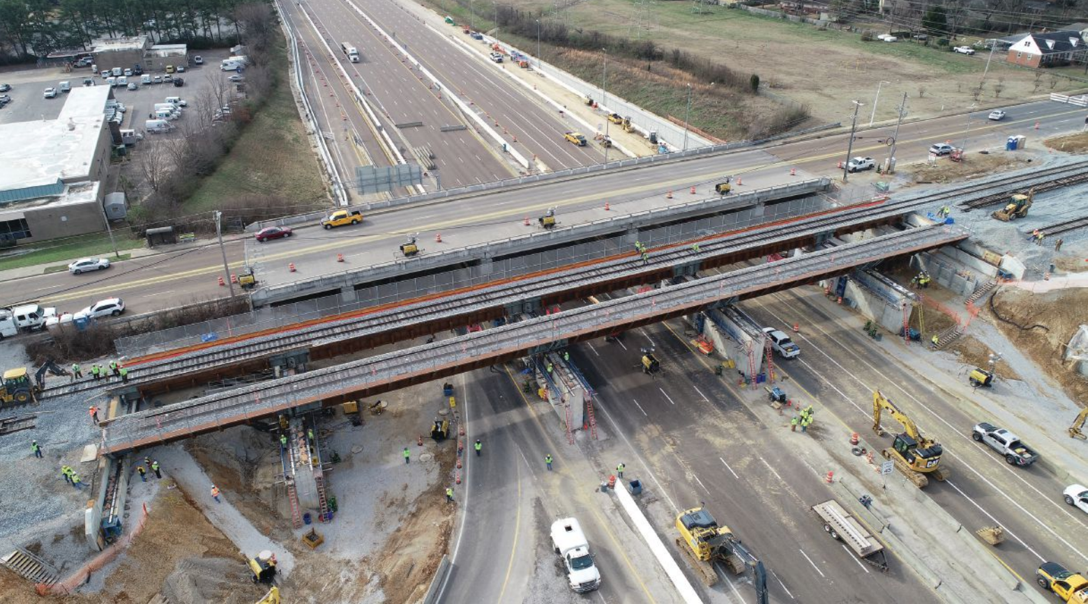
above: Sliding in the second NSR bridge. This replacement railroad crossing comprised a total steel weight of 950 tons and a maximum span of 88 ft.
