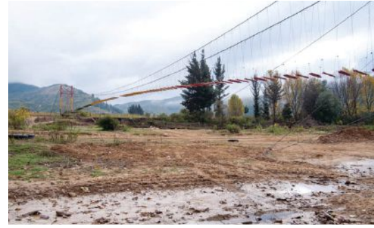
left: The team pulls the main cables as tight as possible before using a winch to set the final tension.
