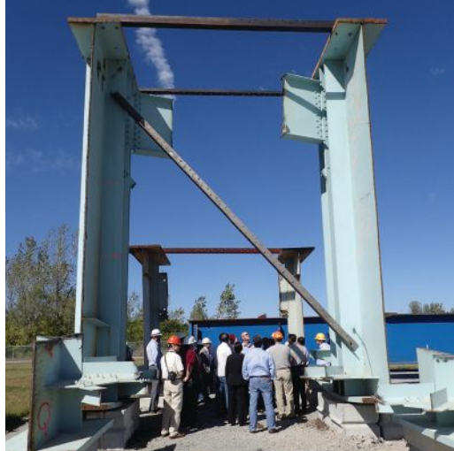
above: A group of engineers is dwarfed by 23-ft-deep girder sections from the Dresbach Bridge—provided by the Minnesota DOT and Ames Construction—which carried I-90 across the Mississippi River between La Crosse, Wis., and Dresbach, Minn.
