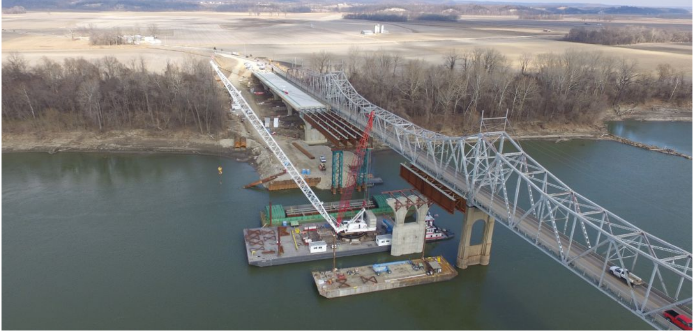
above: Girders were raised using a pair of crawler cranes.
