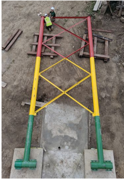
above: Larry O'Connell locates the bracket to stop the columns once they are raised.
