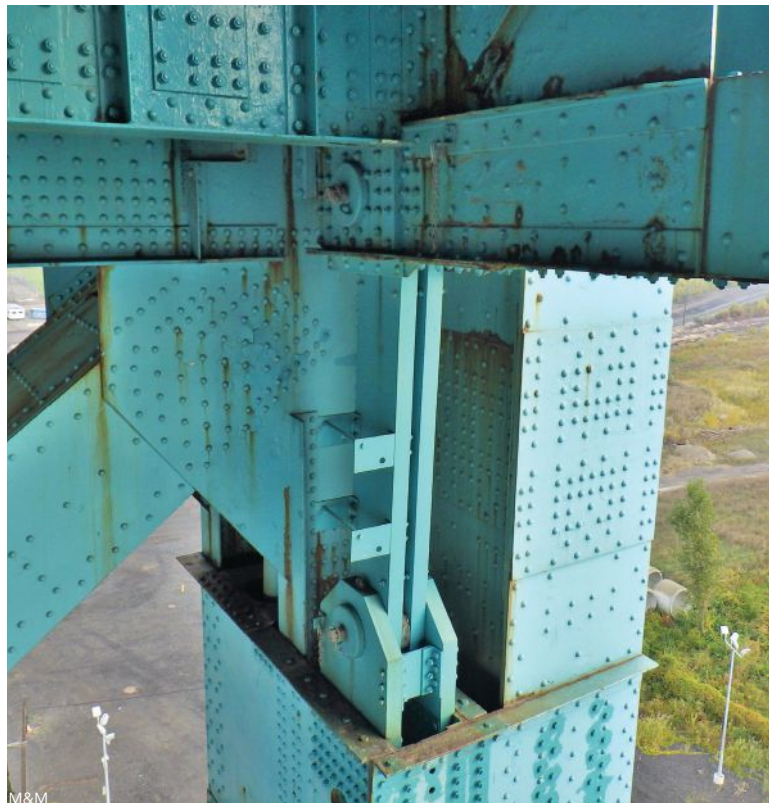
above and below: The rocker link replacement for the Ambassador Bridge. A test lift was used to verify the dead load present at each of the four corners.
