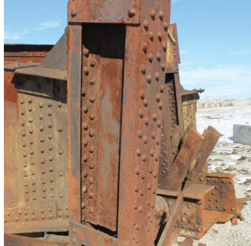
left: A 90-ft-long pony truss obtained from China Township, Mich. The structure contains considerable corrosion damage and includes many welded repairs.
