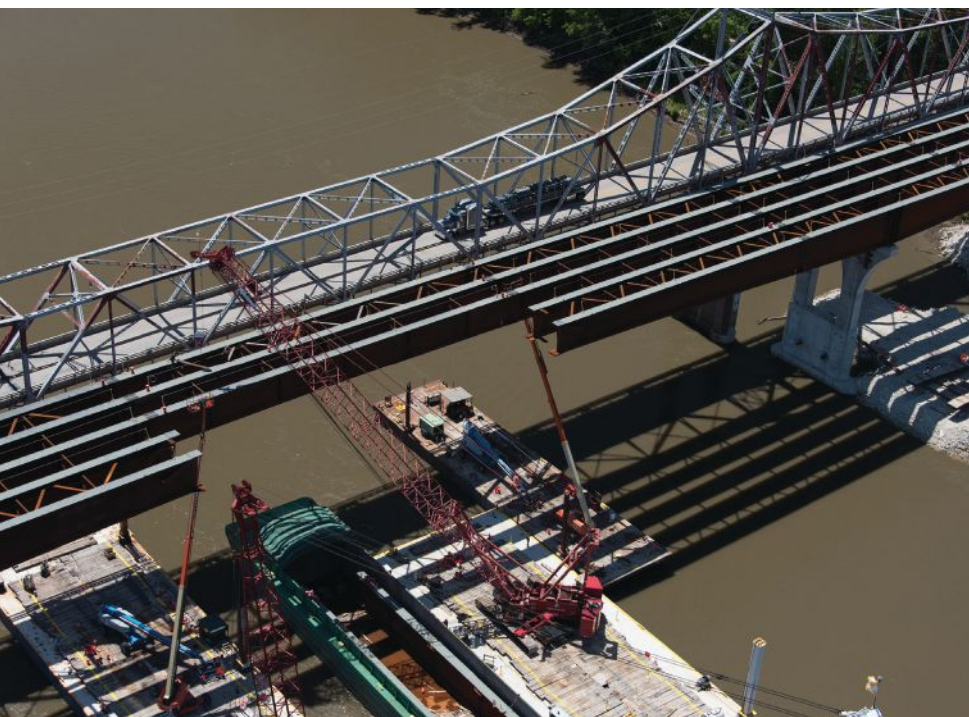
above and left: The bridge's superstructure is made up of 75 individual plate girders whose lengths vary from 100 ft to 140 ft and whose depths range from 18 ft at the support piers to 10 ft, 6 in. at the midspans.
