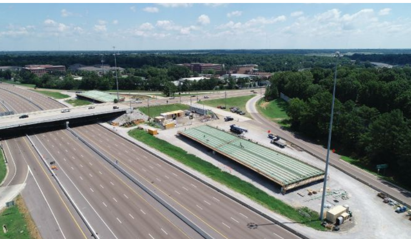
above: Sliding in the second NSR bridge. This replacement railroad crossing comprised a total steel weight of 950 tons and a maximum span of 88 ft.
