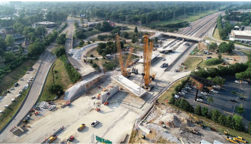
above and below: The Poplar Avenue roll-ins required only two 56-hour closures of I-240, significantly less time than would have been required had the bridges been built in place using concrete.
