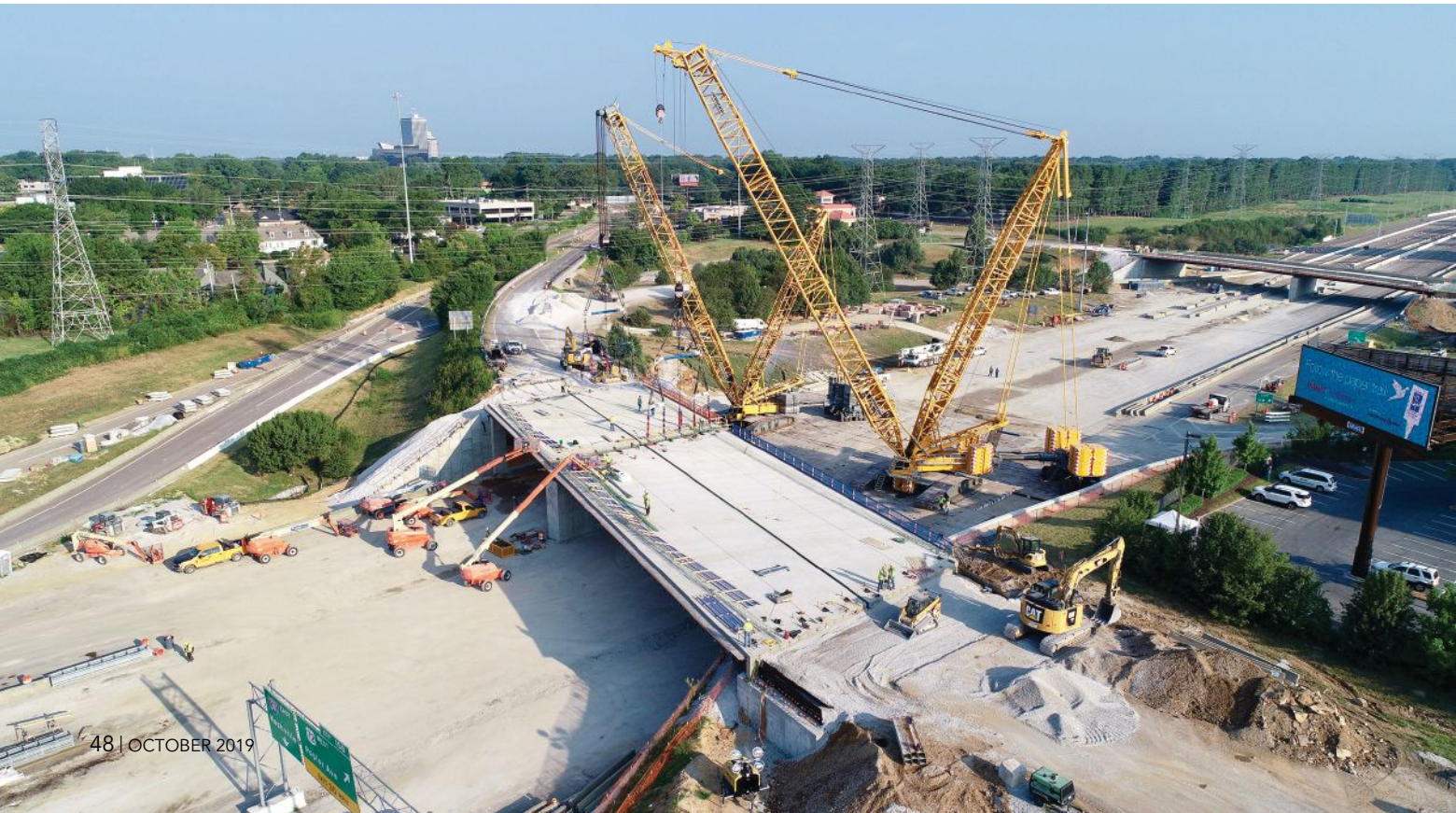
above: On average, opting for steel instead of concrete reduced the depth of the Poplar Avenue structures by about 30% and the weight by more than half. below: After demolishing the existing bridges, the modular superstructure units—with the heaviest being six girders wide, 150 ft long, and 550 tons—were slid into place.
