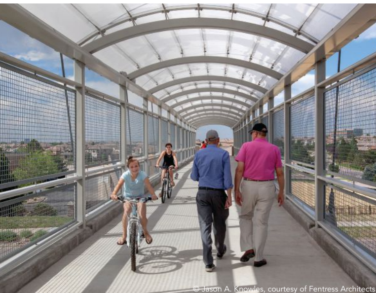
© Jason A. Knowles, courtesy of Fentress Architects
