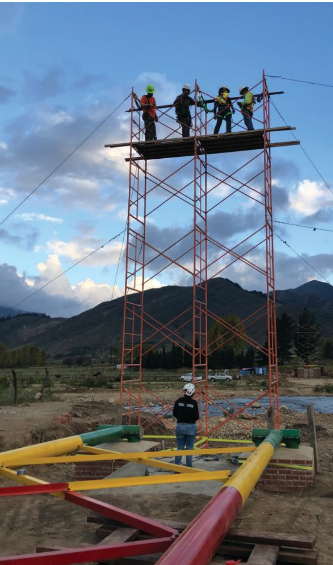
right: Craig Stevens and John Hastings installing cross frames on the towers. The nearly 33-ft-tall towers were made from 10 3/4-in.-OD pipe and L3x3x1/2 cross frames, all connected with 3/4-in. A325 bolts.
