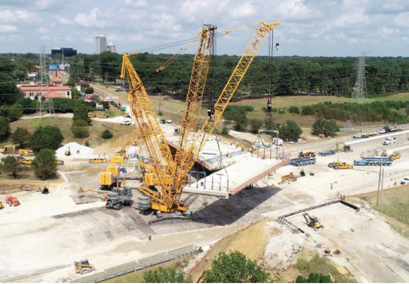
above and below: The Poplar Avenue roll-ins required only two 56-hour closures of I-240, significantly less time than would have been required had the bridges been built in place using concrete.
