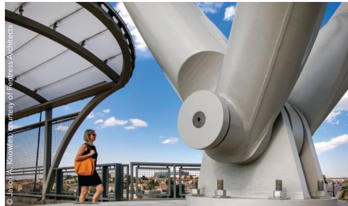
above and left: A steel knuckle at the base of the leaf pylon incorporates a 10-in.-diameter by 4-ft-long stainless steel pin inside a steel sleeve.
