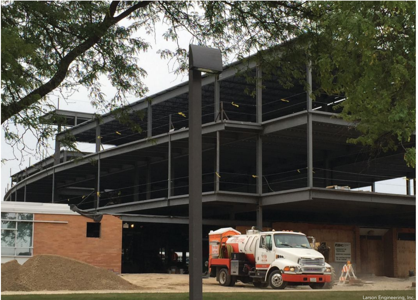
above: Multiple transfer girders using W27×84 and W27×94 members were employed in the second-floor framing.
