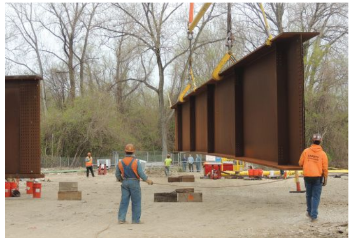
below: Lifting one of the massive plate girders from the ground.
