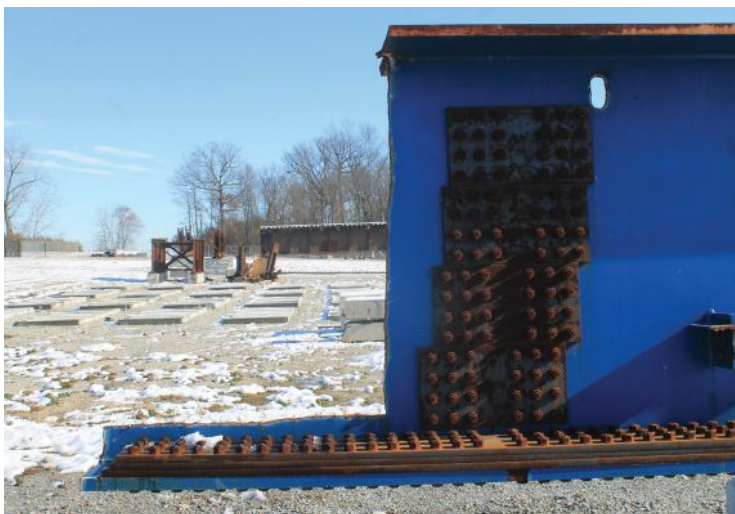
below: A portion of a former fascia girder over an Interstate now illustrates how a bolted girder splice can be used to repair a fracture.
