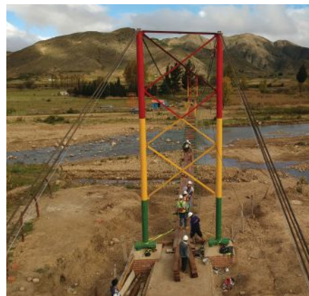
left: Crews working on decking from both sides of the bridge toward the middle.
