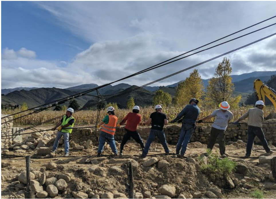
left: The team pulls the main cables as tight as possible before using a winch to set the final tension.
