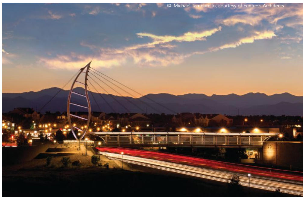
left: For the leaf pylon, the team focused on the sensitivities of the cable and pylon geometry to harmonize steel's efficiency with an artistic design.
