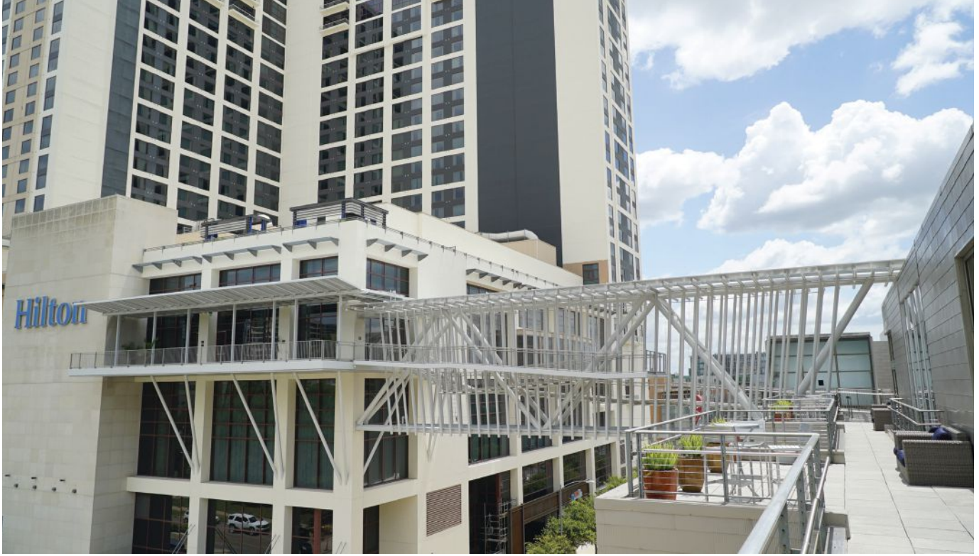
above and left: The balcony and walkway connect to the sixth floor of the Hilton and the third (top) level of the Austin Convention Center, 50 ft above street level.
