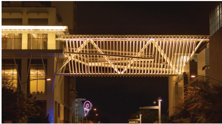
below: The Hilton Overhead Walkway, which uses 90 tons of structural steel, connects the Hilton Austin and the Austin Convention Center above a vibrant section of the city's 4th Street.
