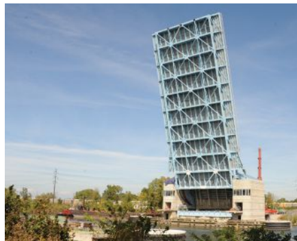
Detroit's Fort Street Bridge over the Rouge River, a 2018 Prize Bridge Award winner.
