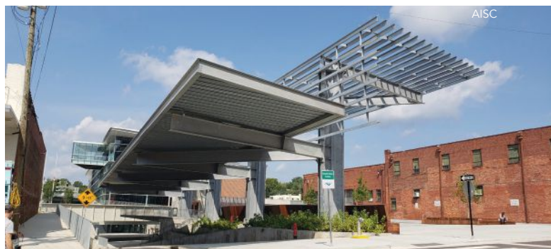
below: The galvanized plaza canopy serves as a dramatic entrance.
