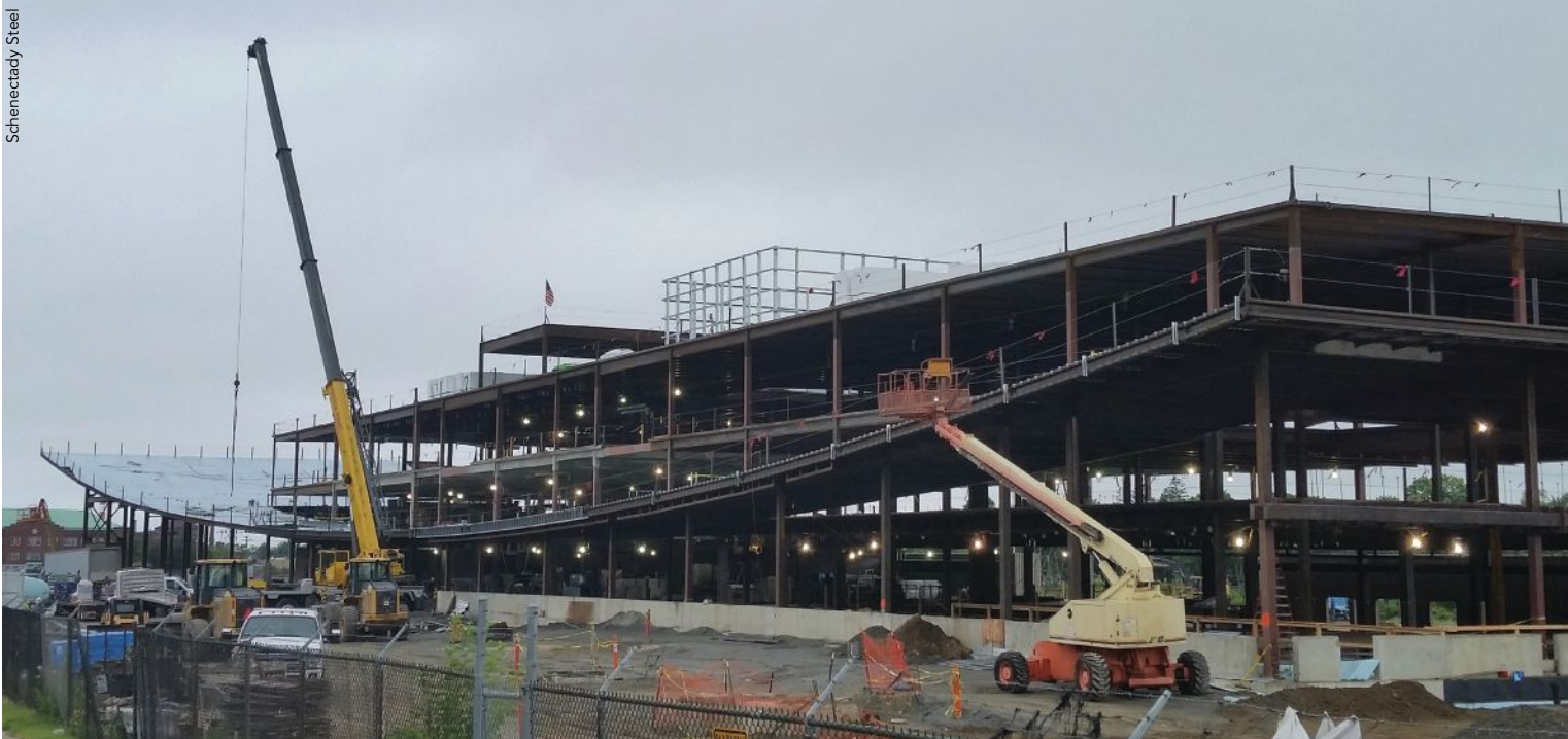
below: The curved portion of the roof combines form and function, incorporating the wide range of roof deck heights required by a high school auditorium, classrooms, and office space while at the same time creating an opportunity for a signature architectural feature.
