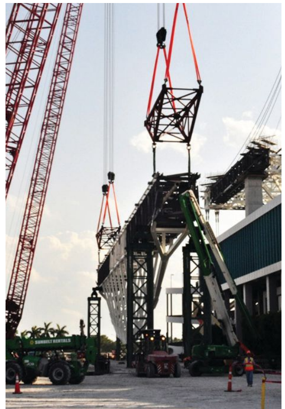
A spreader beam (above) and a multi-crane lift using triangular frames (right) were employed to erect the Hard Rock Stadium Shade Canopy in Miami Gardens, Fla. (The project was a 2018 AISC IDEAS 2 Award winner. See the May 2018 issue at www.modernsteel.com .)
