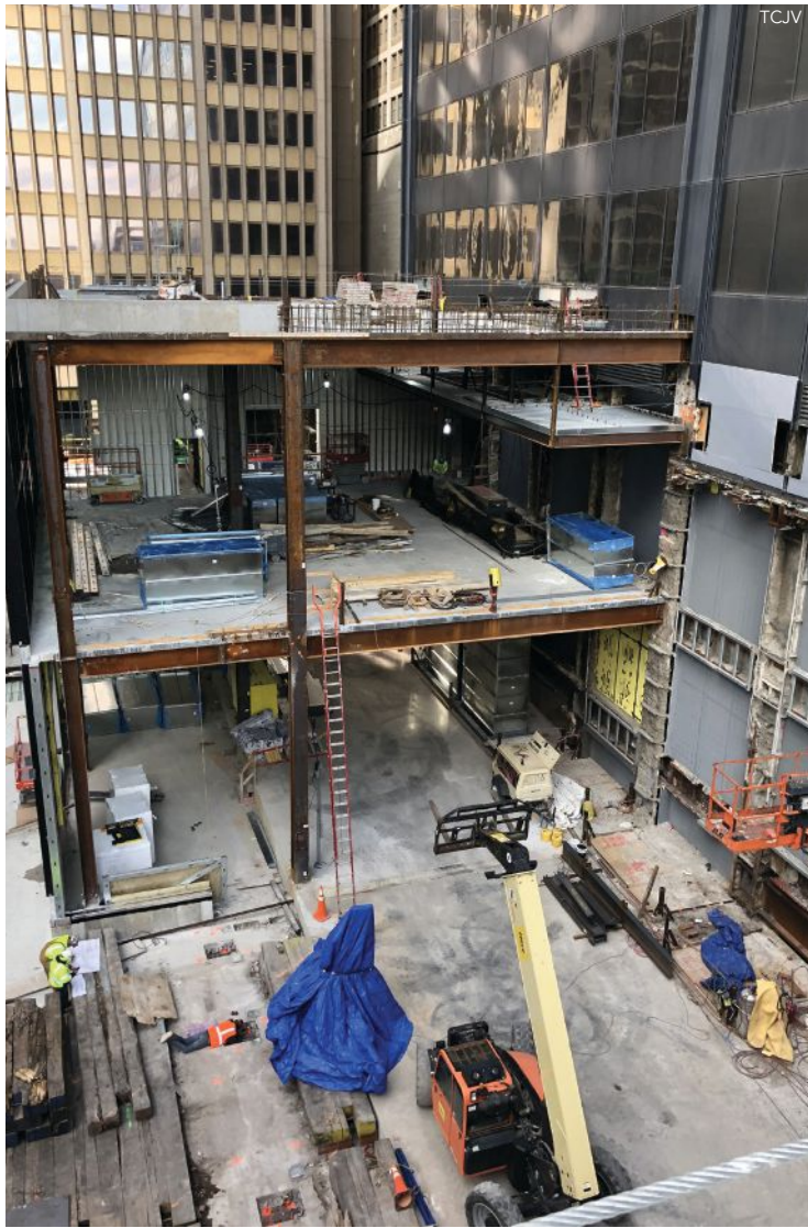
above and below: Framing for the new Wacker entrance. To see the below model "dance," see the Project Extras section at www.modernsteel.com .
