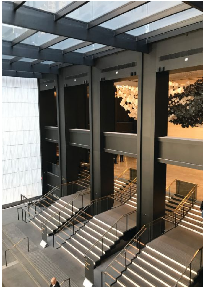
above: An AESS glazed structure encloses the Wacker entrance and permits a straight line of sight from street level to the top of the 110-story tower.
