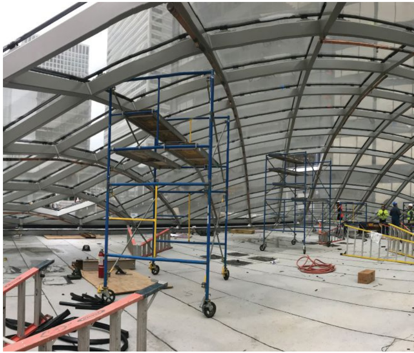
above and below: An AESS support system in the form of a lightweight, undulating grid shell caps off the new "Catalog" atrium, named as an homage to Sears.
