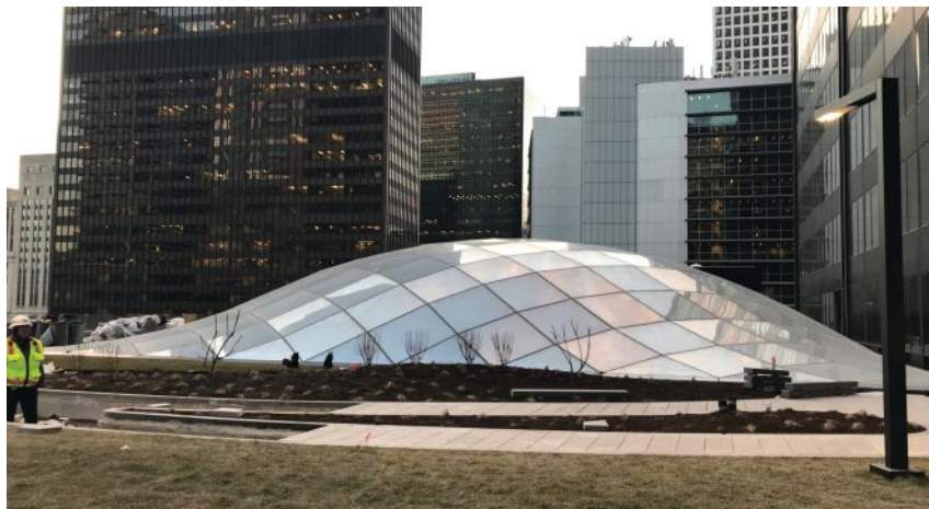
above and below: An AESS support system in the form of a lightweight, undulating grid shell caps off the new "Catalog" atrium, named as an homage to Sears.
