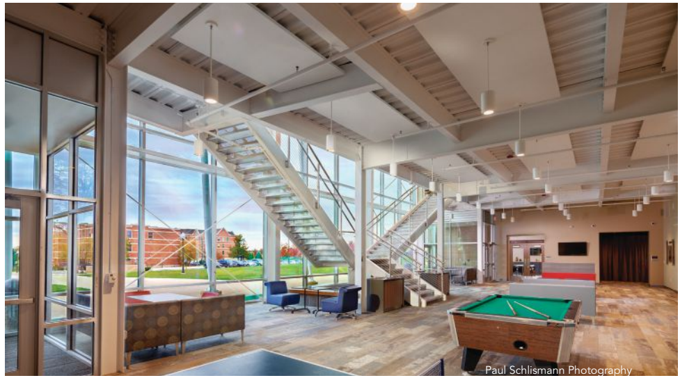
above and below: The curtain wall exposes a steel-framed stairwell that splits into two segments as it rises between the first and second floors.
