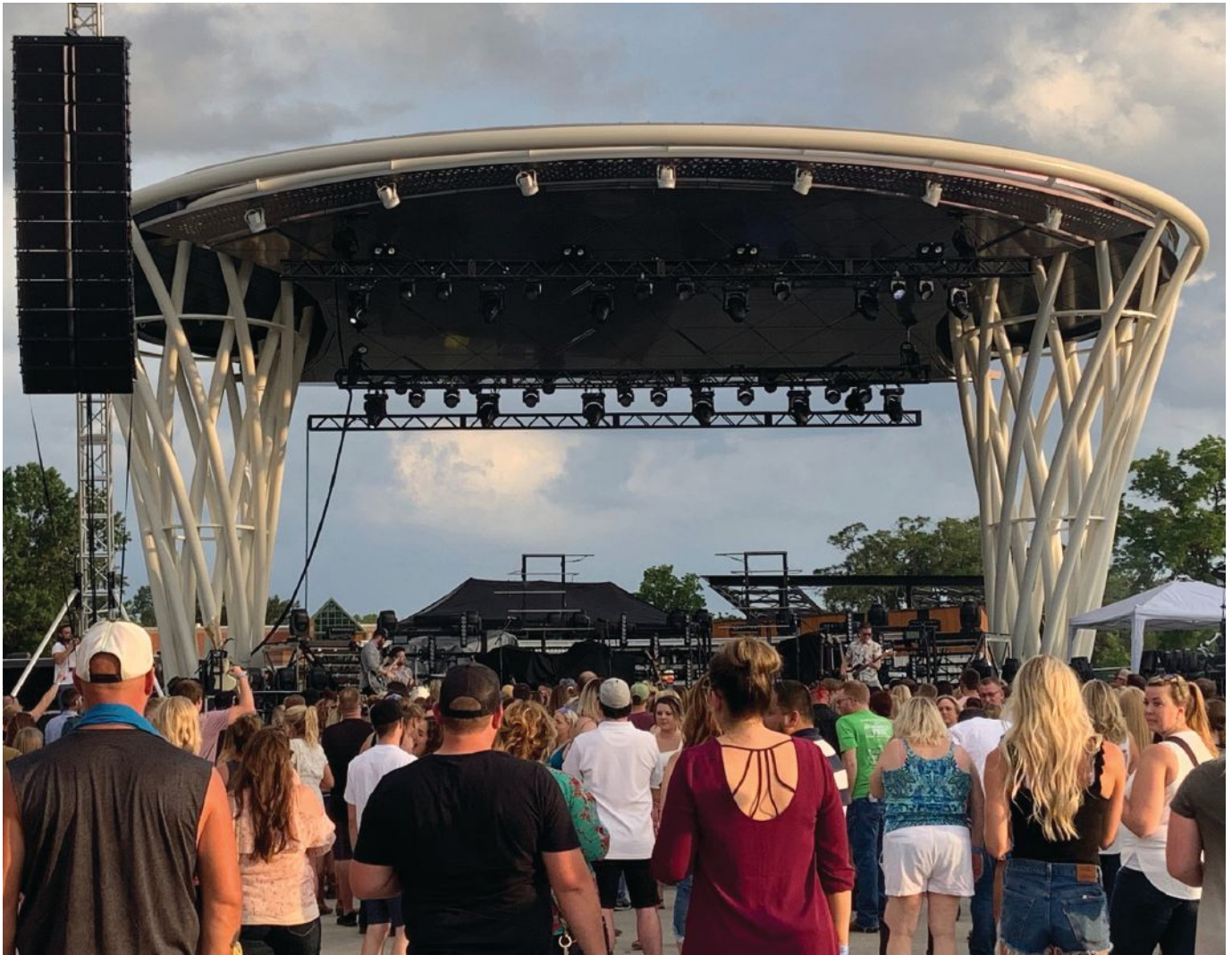
above and right: The complex, curved steel column assemblies are a natural response to the local environment, inspired by the form of an oak tree. Each weighs 13.5 tons.
