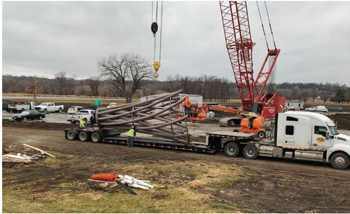
above: Transporting the bottom half of one of the tree column assemblies to the site.
