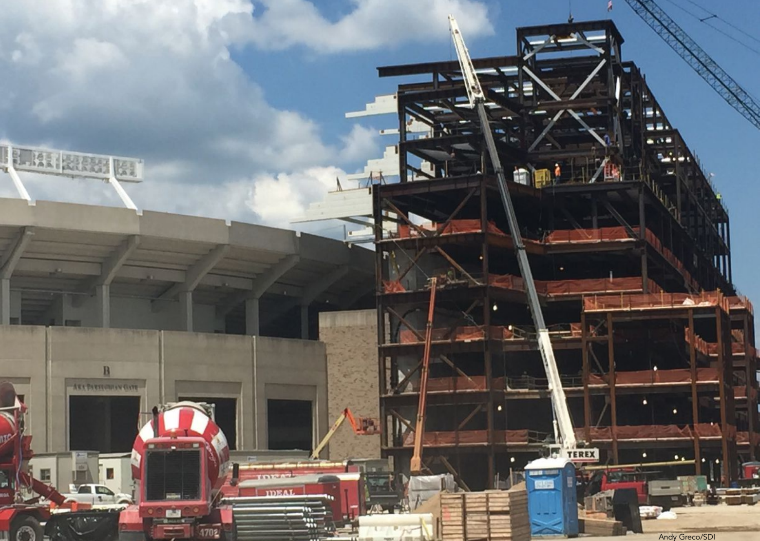
below: The original press box was demolished following Notre Dame's final game of the 2016 season to allow the new cantilever trusses to take their place.
