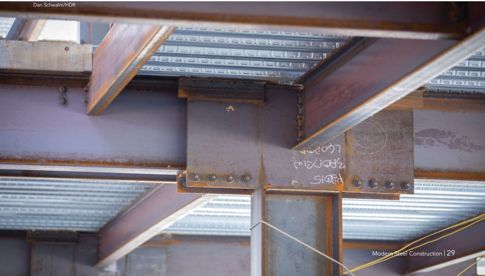
above: As this was Nebraska's first SidePlate system, steel fabricator Paxton and Vierling Steel (PVS) built a mock-up of a SidePlate connection in its shop to review constructability issues.
