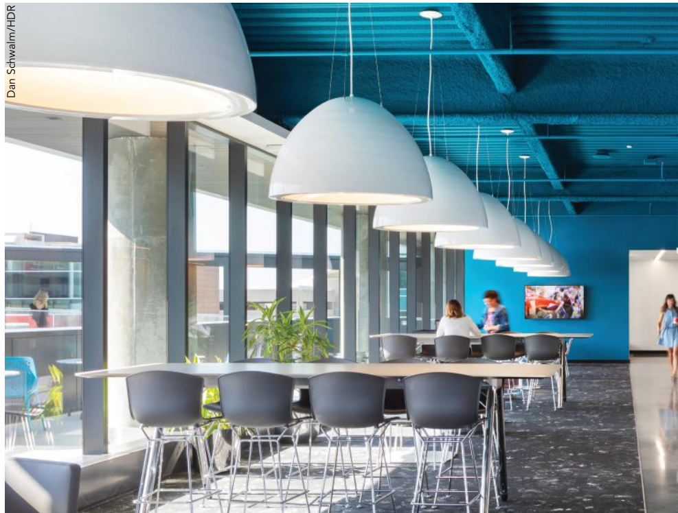
below: Exposed beams are protected with spray-applied fireproofing topped with paint.
