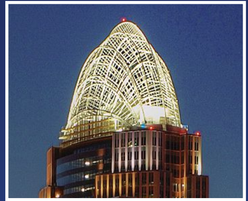
2012 IDEAS 2 Merit Award - 133 tons of 16" pipe curved for the Rooftop Tiara of the Great American Tower at Queen City Square. Cincinnati, OH
