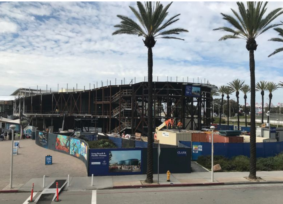
above and below: The framing for the addition used 350 tons of structural steel and 4,831 connection bolts to hold it all together—all delivered from North Dakota to Long Beach in 30 truckloads.
