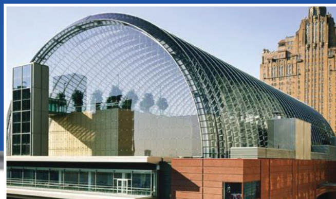
2003 IDEAS 2 National Winner - 300 tons of 5" square tubing curved 45° off-axis for the Kimmel Center. Philadelphia, PA
