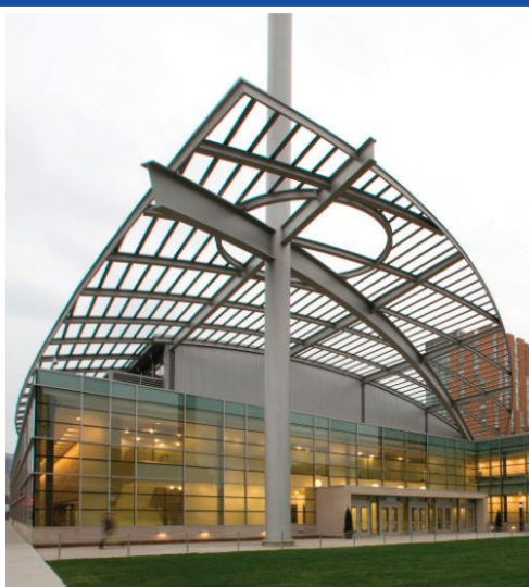
2010 NCSEA Award Winner - 200 tons of beams, channels and angle for the roof of the University of Illinois at Chicago Forum. Chicago, IL
