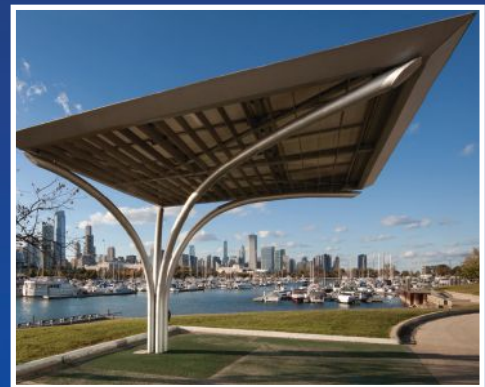
2013 IDEAS 2 Merit Award - 3600 pounds of pipe each curved with multiple radii for a solar canopy to recharge batteries on electrical vehicles. Chicago, IL
