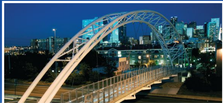
2007 NSBA Special Purpose Prize Bridge Award - 152 tons of 18" pipe curved in our Kansas City plant for the Highland Bridge. Denver, CO
